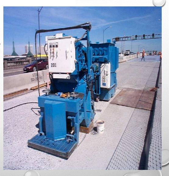
Shot Blasting will remove 15 to 40 mils of concrete off the surface by propelling steel shot onto the floor. This provides for a light to heavy textured sidewalk finish. Shot Blasting will blast patterns that range from 6" to 30" in width. This preparation process creates an ideal bonding profile for thick mil coatings (25 mils and above).
