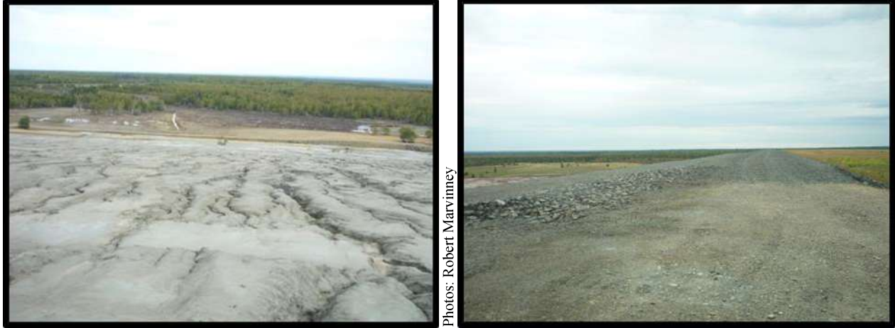
Tailings dam at a legacy mine. Left picture looks directly down the slope of the dam, built from tailings, showing significant gully erosion. Right picture shows the top of the dam structure, with rock armoring along the left and stabilized tailings to the right. ( Brunswick No. 12 mine, New Brunswick. )
