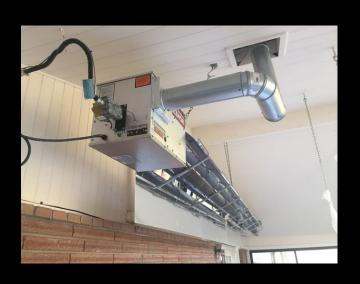
Emergency Switches & TC-1's are NOT required on space heating appliances
