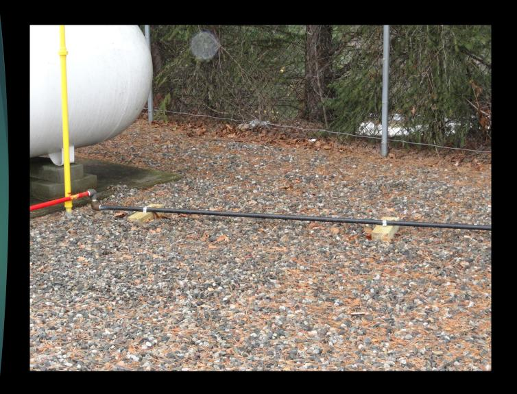
Aboveground piping shall be protected from vehicle damage
