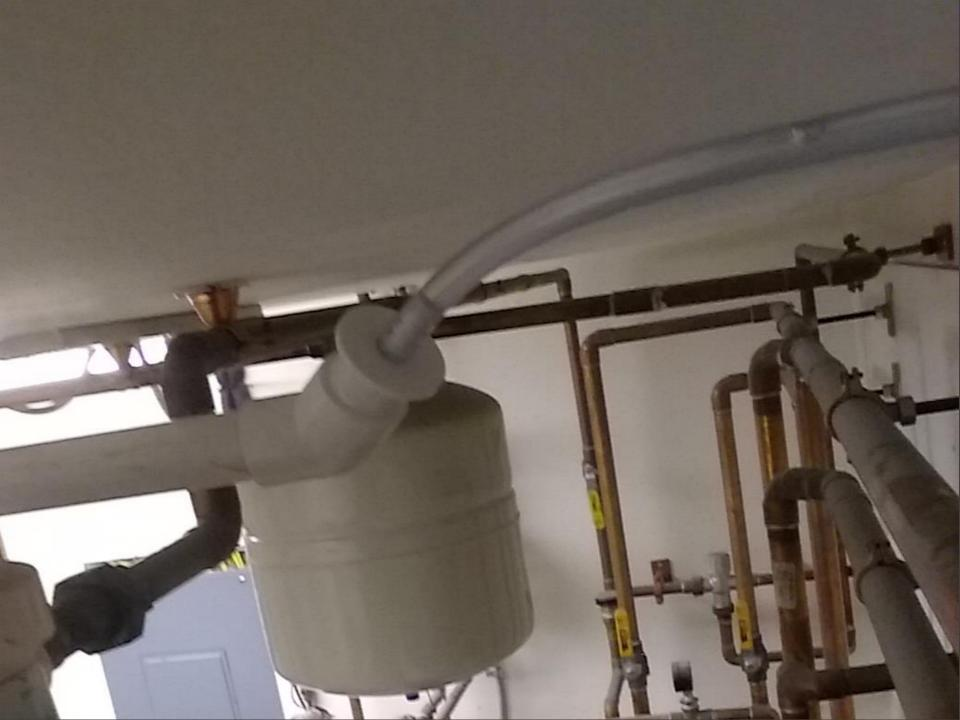
The gravity condensate drain (waste pipe) must consist of a corrosion resistant material
