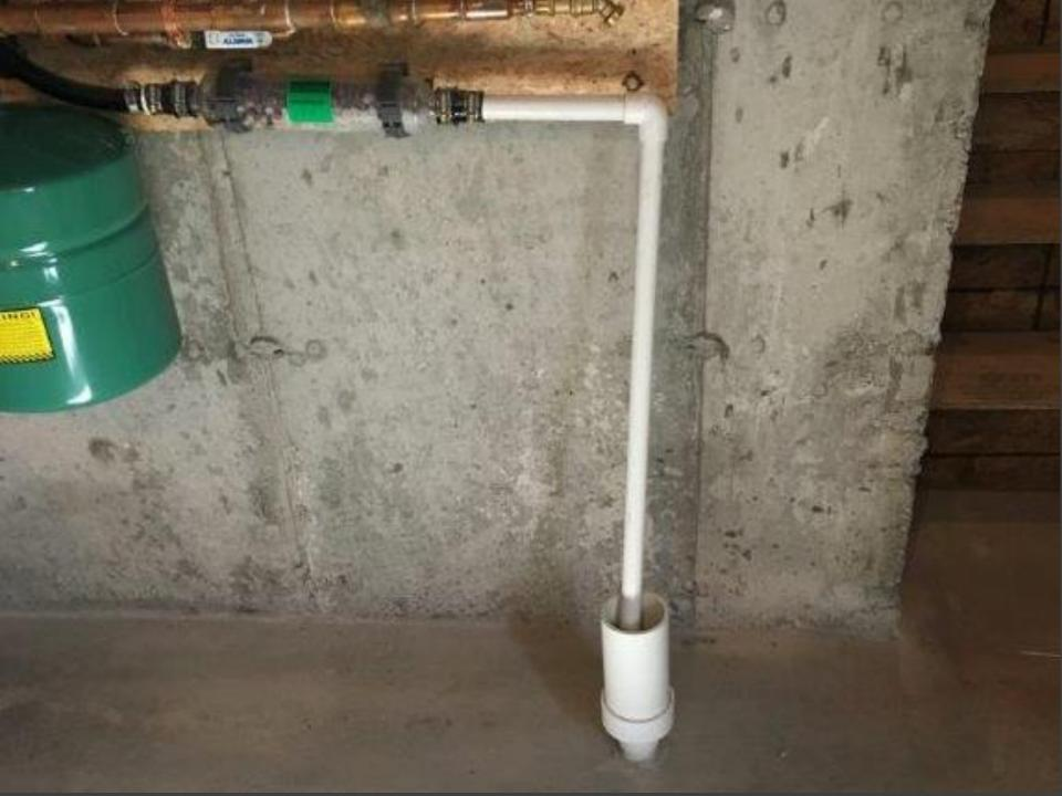
Condensate from fuel fired appliances must be neutralized prior to disposal.
