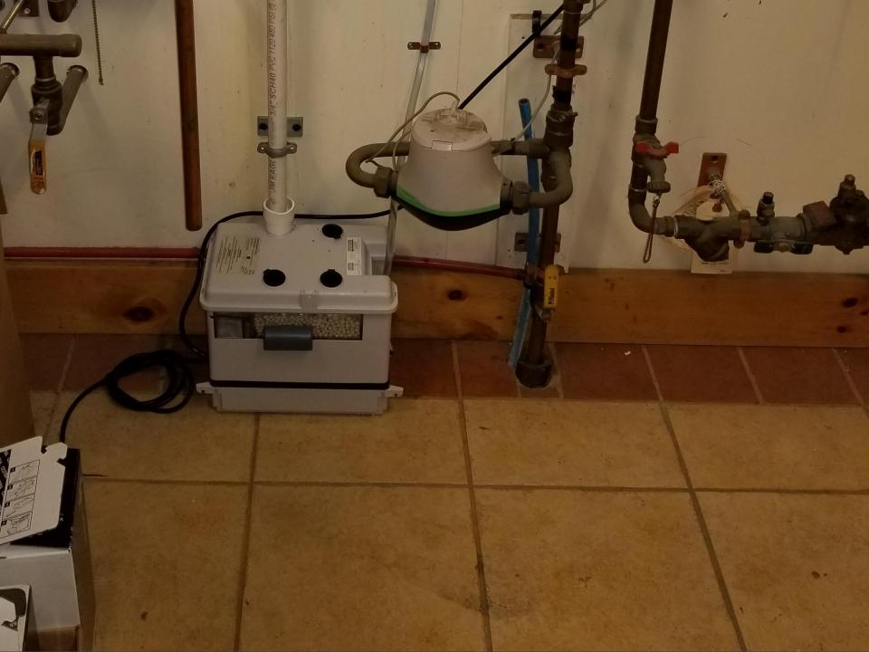
The use of copper tubing for condensate disposal is prohibited.
