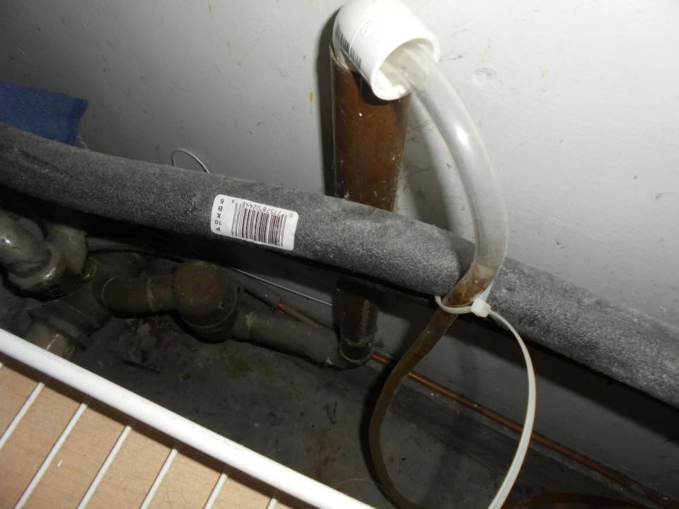
The waste pipe must maintain a slope of 1/8" per foot minimum towards the approved plumbing receptacle. In single appliance installations, the waste pipe must be sized according to appliance manufacturers instructions.
