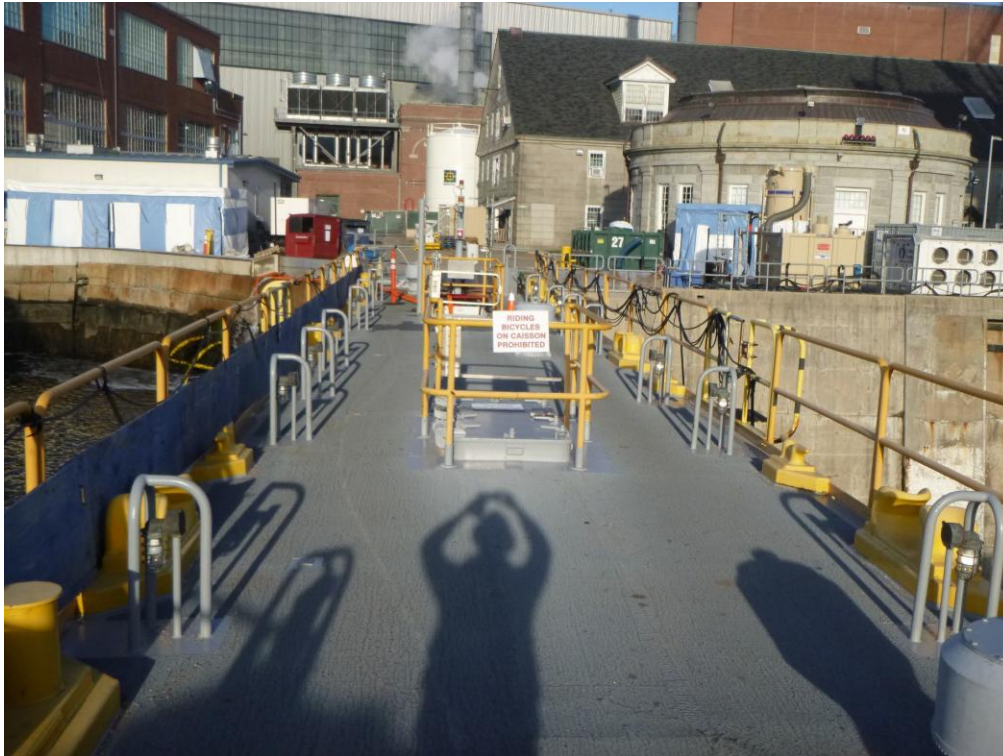
Figure 4. DD2 Caisson Gate Weather Deck Looking West (Approved for Public Release; Photo by Collins Engineers, Inc.)
