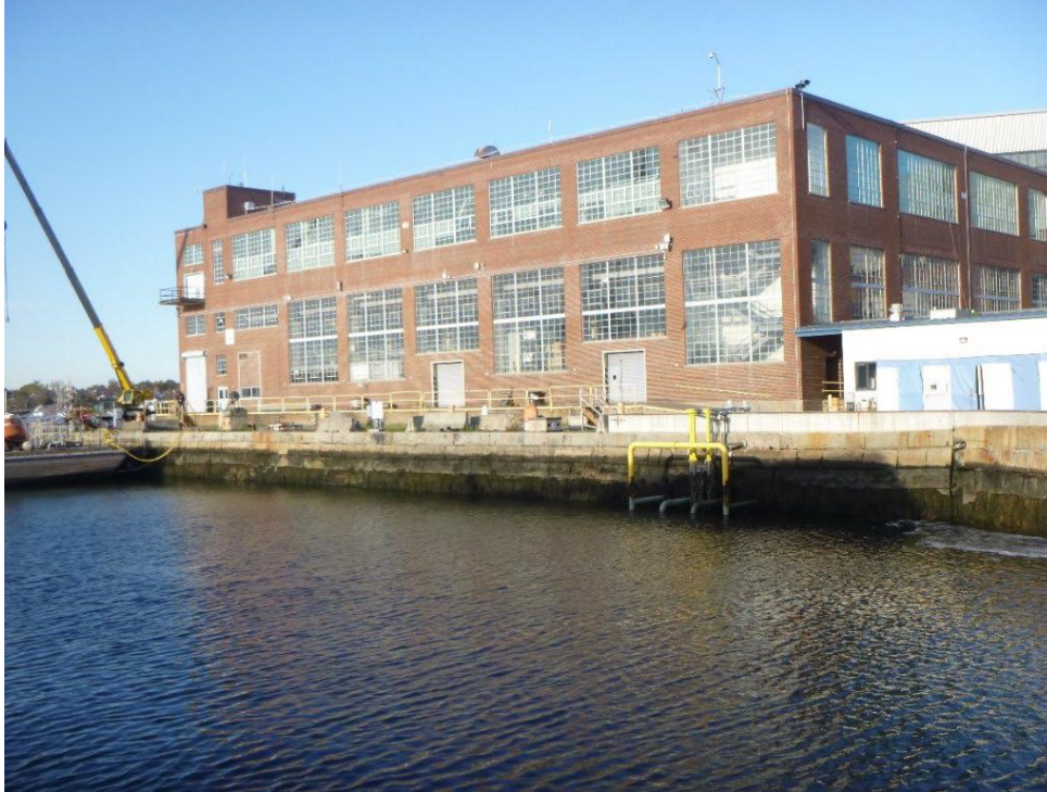
Figure 2. Figure 1: Berth 5 looking west toward Building 238 (Approved for Public Release; Photo by Collins Engineers, Inc.)
