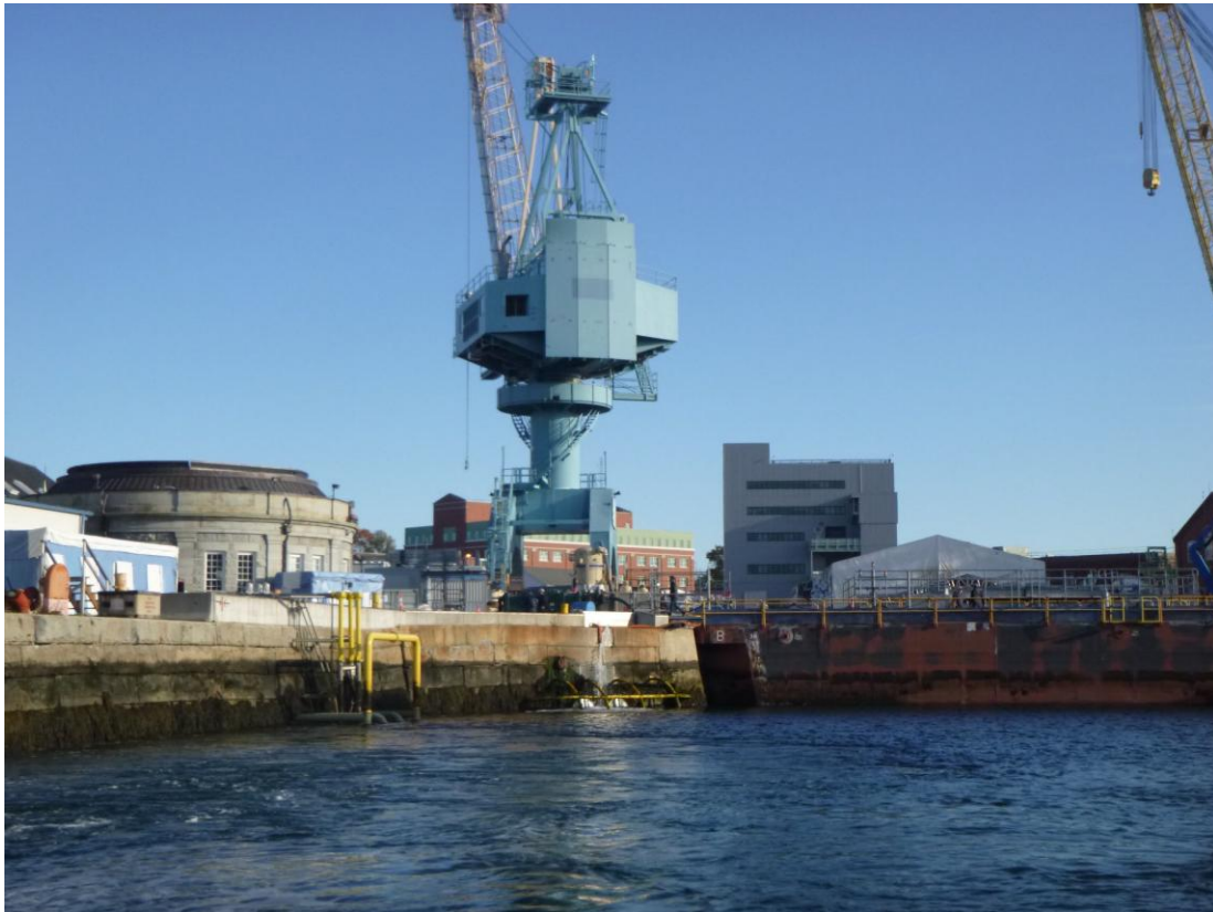
Figure 1. DD2 Caisson Gate Elevation Looking North (Approved for Public Release; Photo by Collins Engineers, Inc.)
