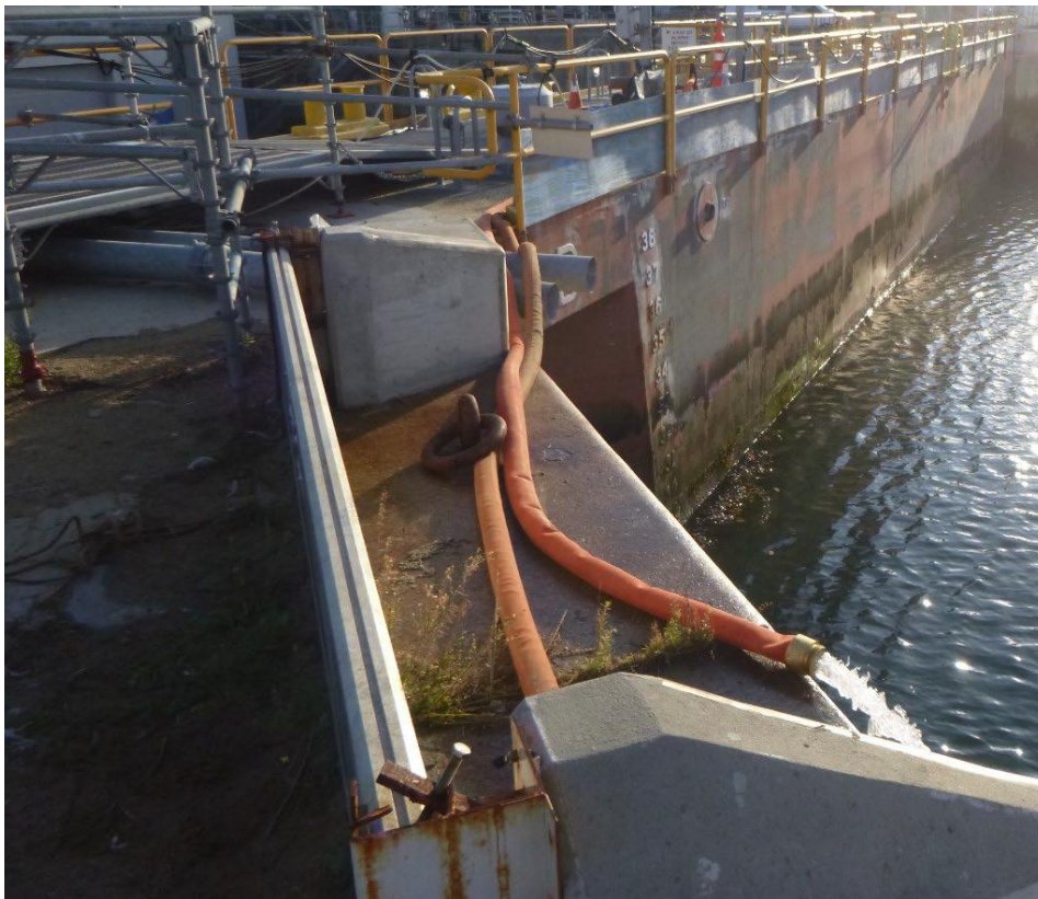
Figure 3. Top of Berth 5 at Dry Dock 2 Caisson (Approved for Public Release; Photo by Collins Engineers, Inc.)
