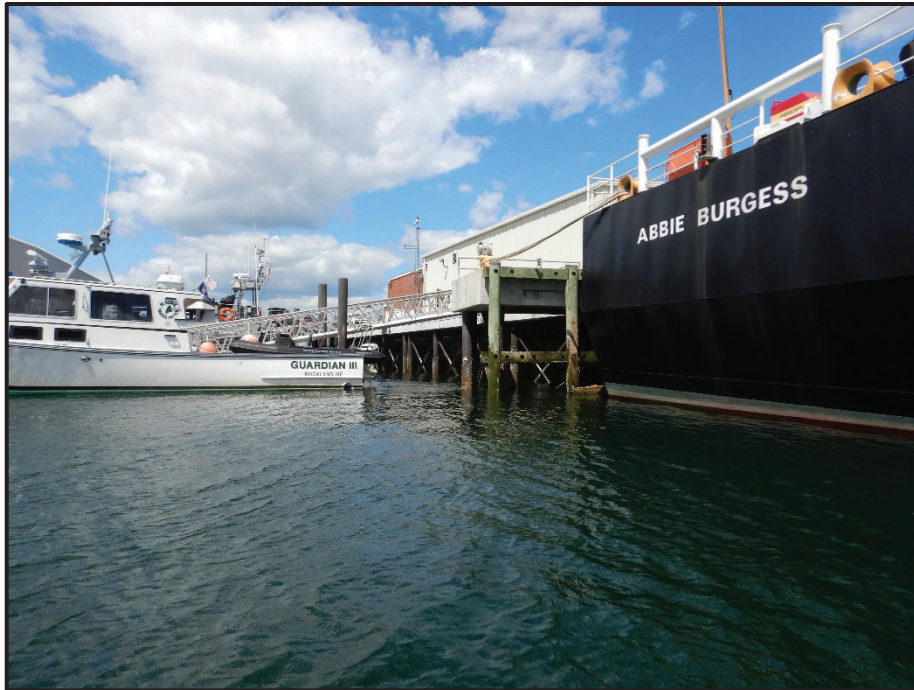
Overall View of West Wharf, Looking Northeast
