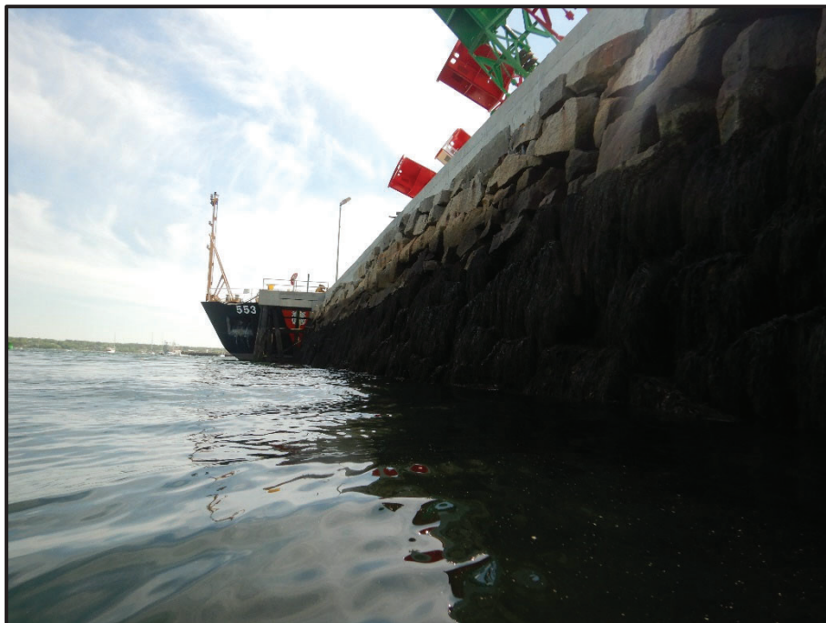
Overall View of East Quay Wall, Looking South
