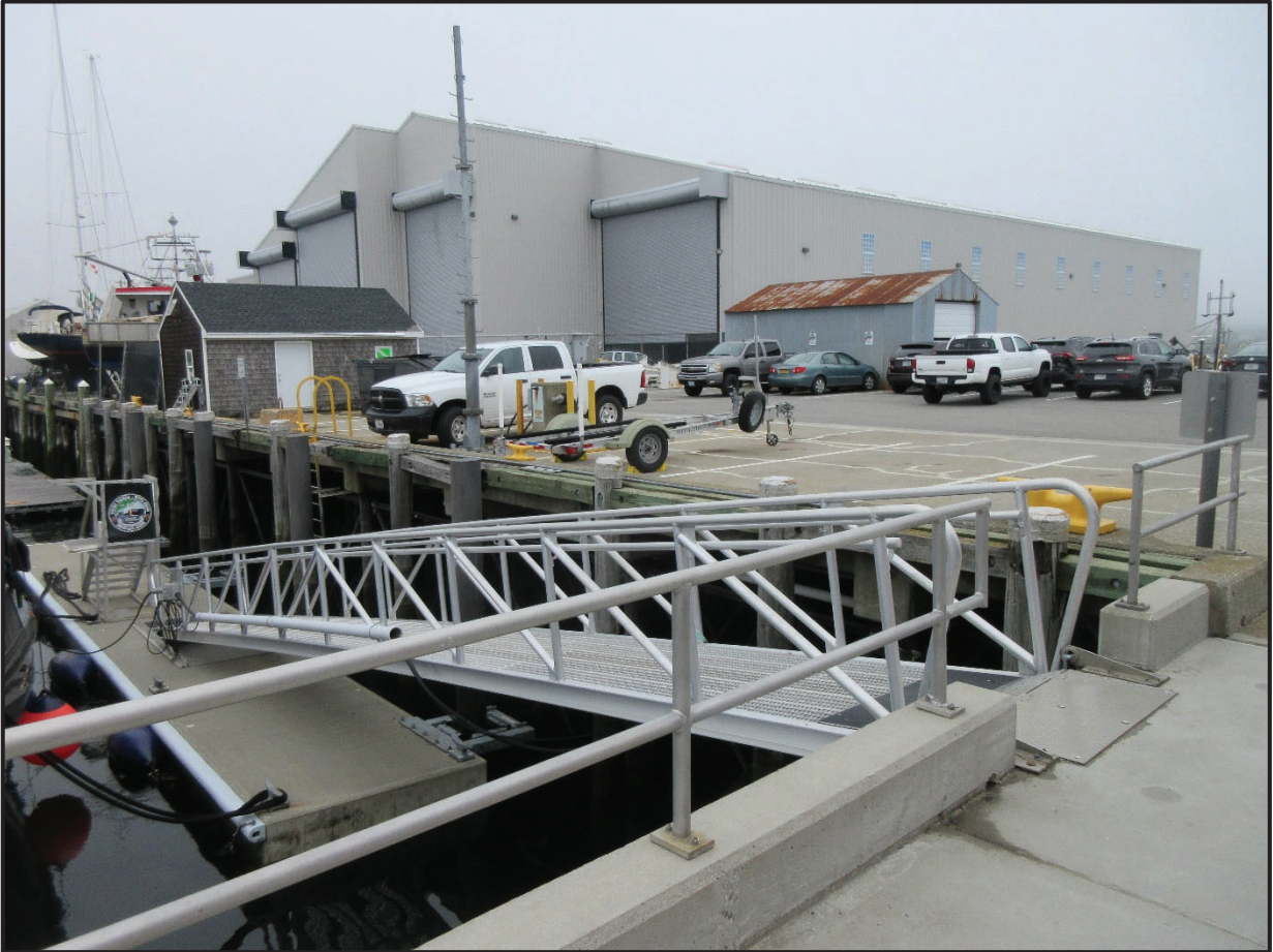
Overall view of the Southwest Wharf, Looking Northwest
