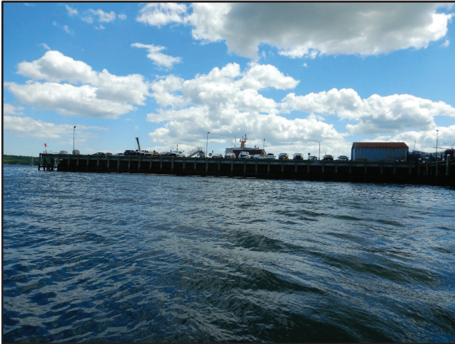
Overall View of the North Wharf, Looking South
