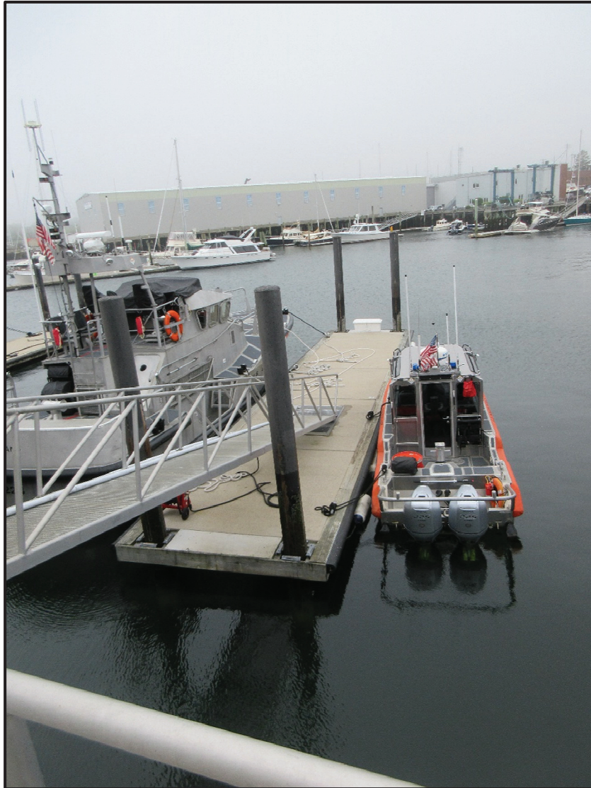
Overall View of the Middle Floating Dock, Looking West
