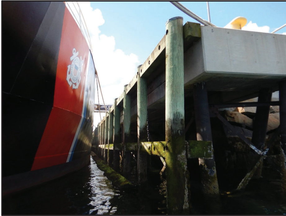
Overall View of the Southeast Wharf, Looking West
