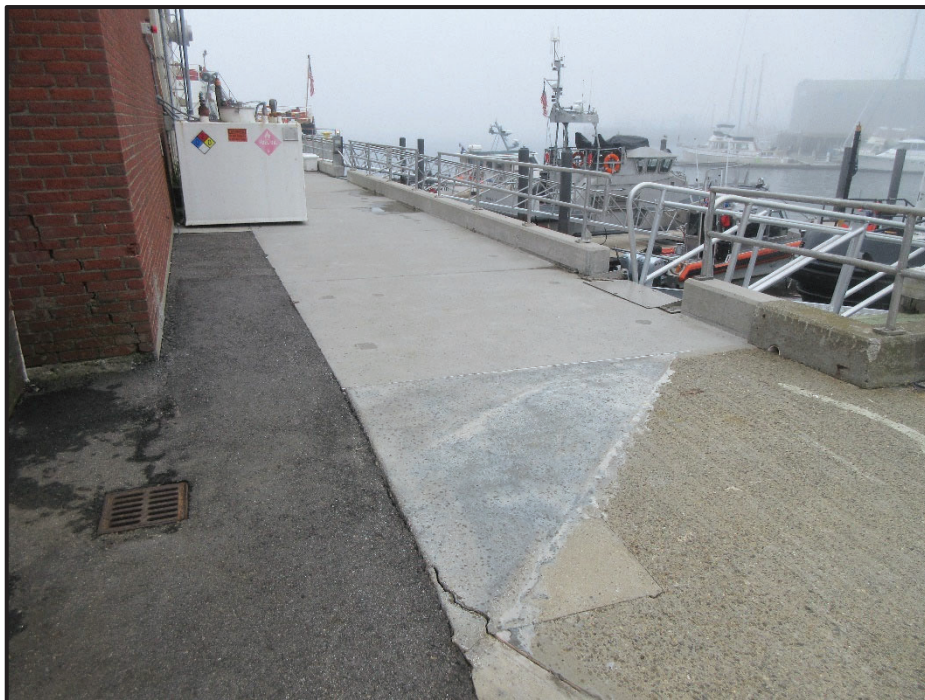
Overall View of the West Wharf, Looking Southwest
