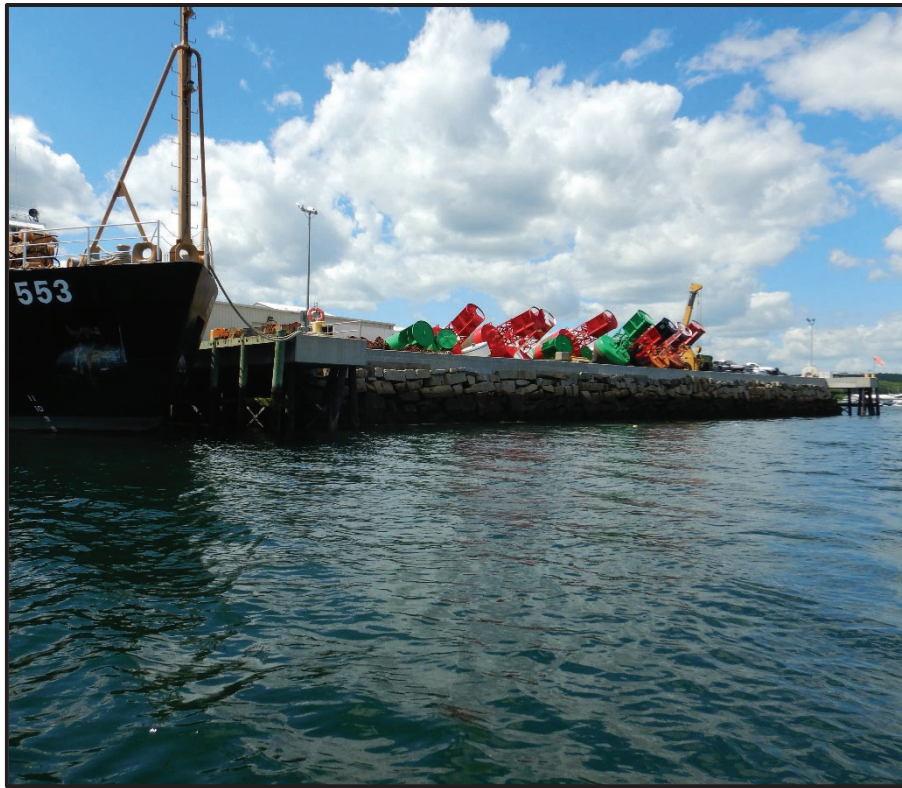
Overall View of the East Quay Wall, Looking Northwest
