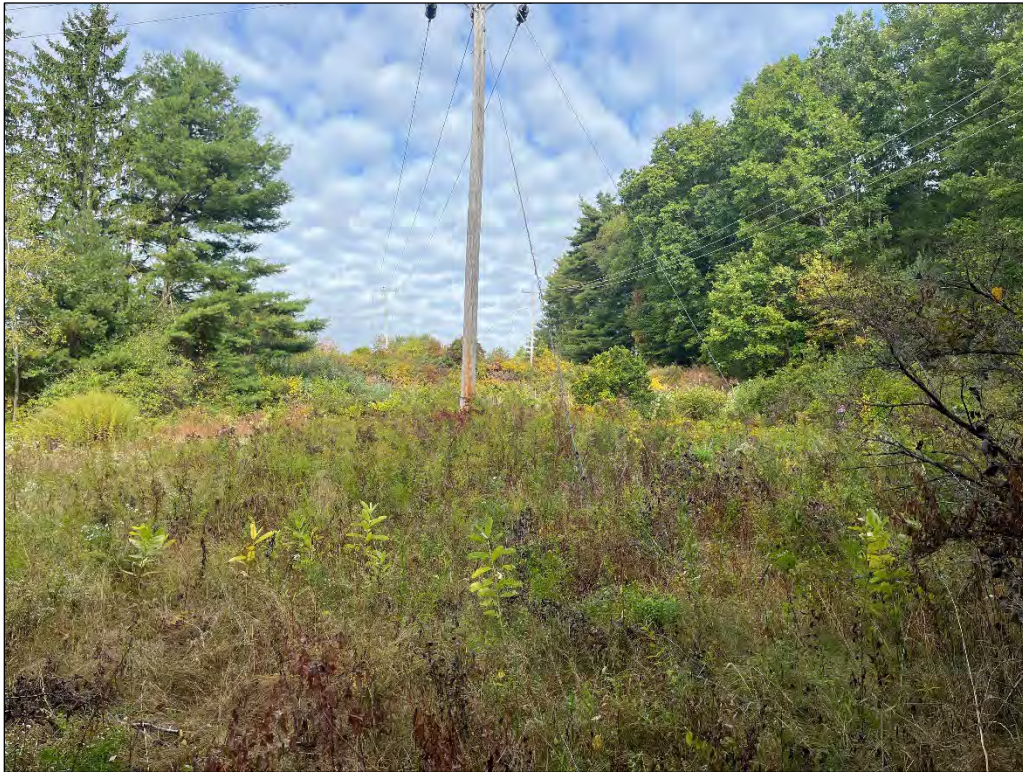
Figure 12. View northwest of SA-03 near Bolt Hill Road.
