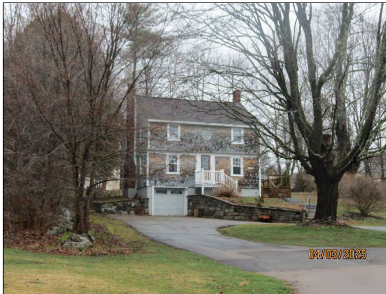
Figure 35. View of 1048 State Road, facing northwest.
