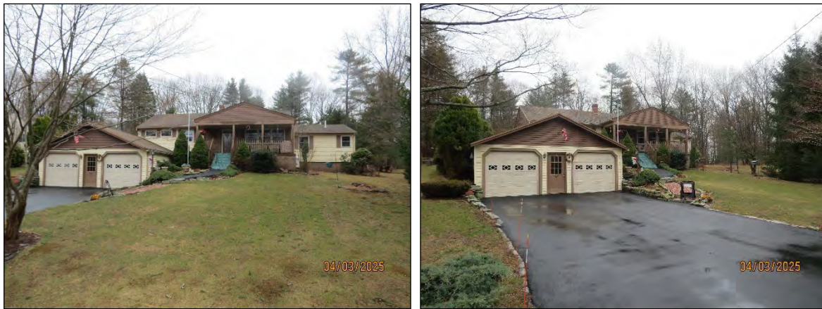
Figure 43. View of 17 Leach Road, facing southeast (left) and facing south (right).
