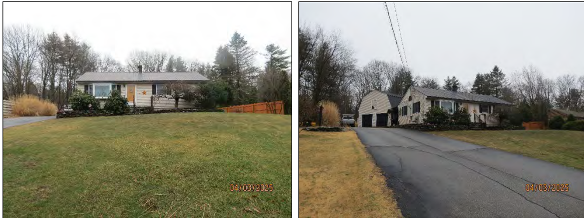
Figure 41. View of 13 Leach Road, facing southeast (left) and facing south (right).
