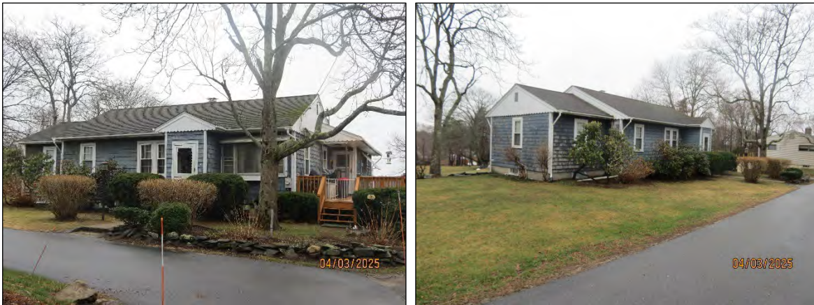
Figure 33. View of 8 Hickory Lane, facing southeast (left) and facing south (right).
