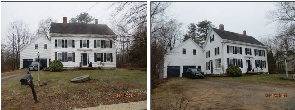
Figure 39. View of 1019 State Road, facing southwest (left) and facing west (right).
