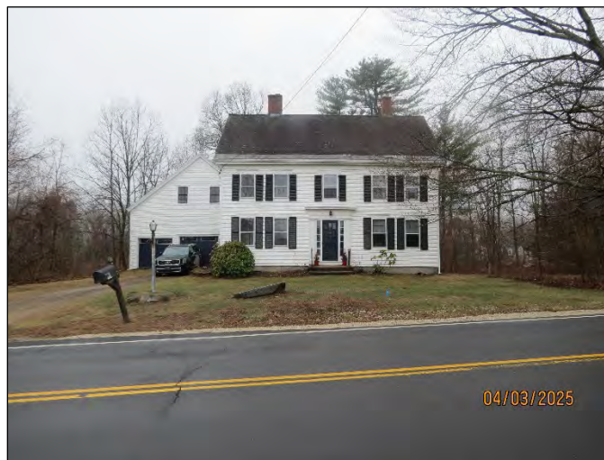
Figure 7. View of 1019 State Road, an example of the Colonial Revival style.
