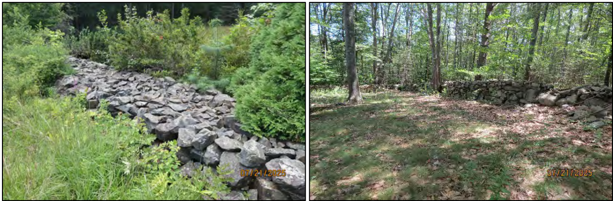
Figure 3. Northeastern retaining wall, facing north (left); southeastern boundary wall, facing northeast (right).
