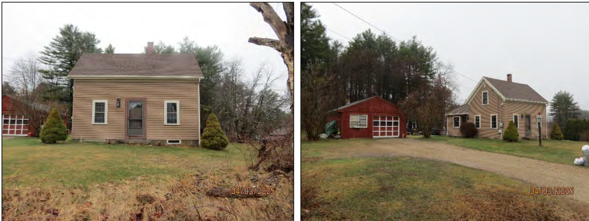
Figure 21. View of 243 Bolt Hill Road, facing northwest (left) and facing north (right).
