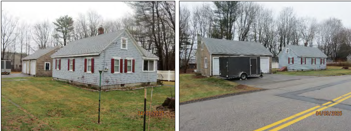
Figure 15. View of 226 Bolt Hill Road, facing east (left) and facing south (right).
