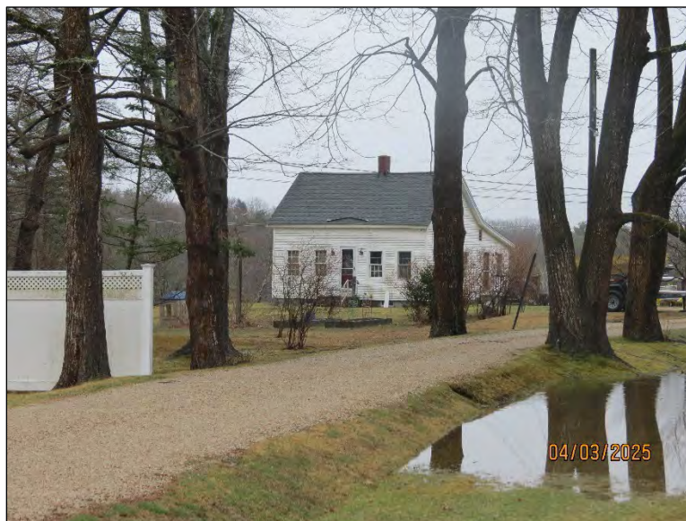
Figure 13. View of 224 Bolt Hill Road, facing southeast.
