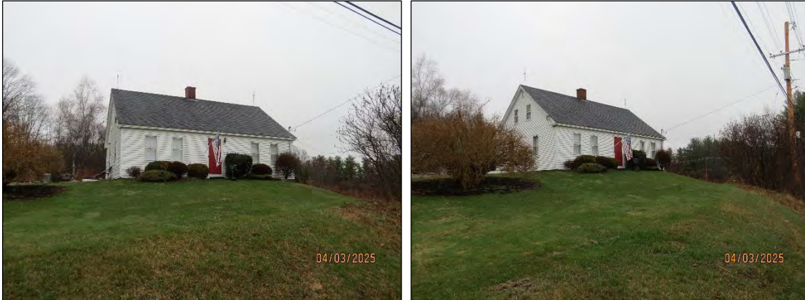
Figure 29. View of 325 Bolt Hill Road, facing northwest (left) and facing north (right).
