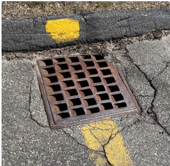
Storm drain on Tuttle Road.
