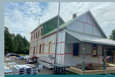
Old Bigelow Train Station Under Renovation
