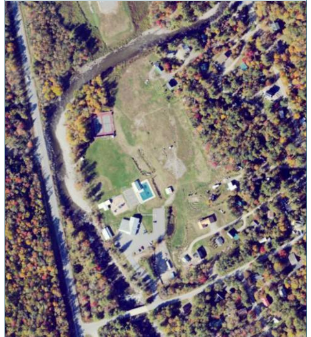
Town Park and Town Office general area.
