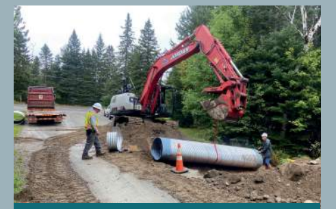
Outdoor Center Access Road - Installing Culverts
