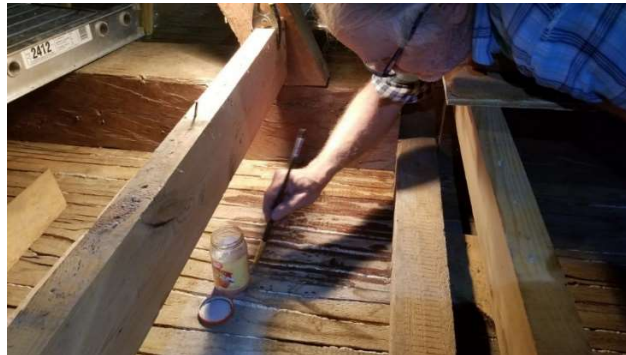
Trompe l'oeil ceiling repair, Union Meeting House, Readfield, 2020
