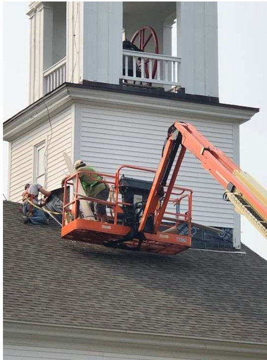
Replacing tower box siding at the Bell Hill Meeting House, Otisfield in 2021. Photograph by Ken Bartow.
