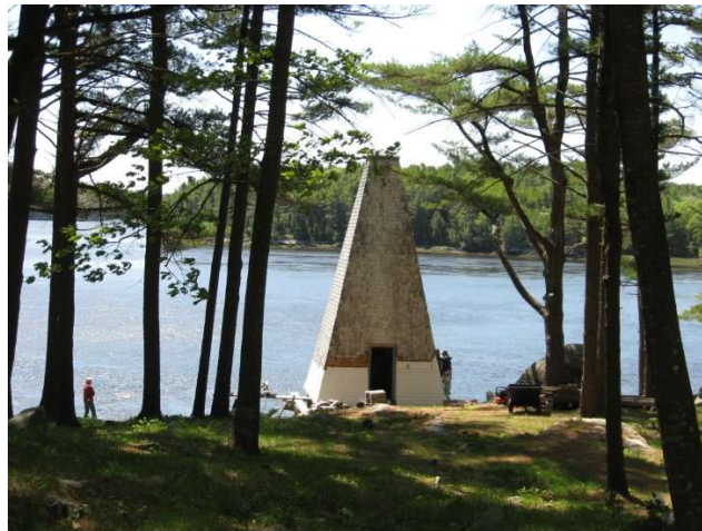
Fiddler's Reach Fog Bell Tower, Arrowsic, 2009, MHPC
