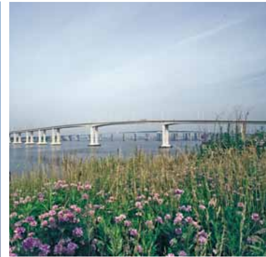
Victory Bridge, NJ [FIGG]
