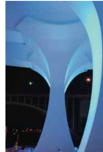
New I-35W Bridge, MN [FIGG]
