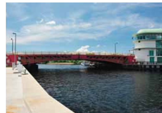
SR-7/NW 5th St. Bridge over Miami River, FL [H&H]
