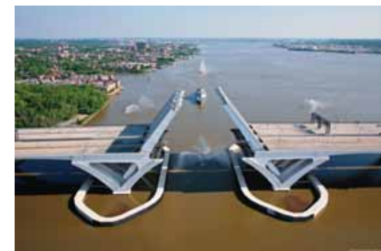
Woodrow Wilson Memorial Bridge, Washington, DC [H&H]
