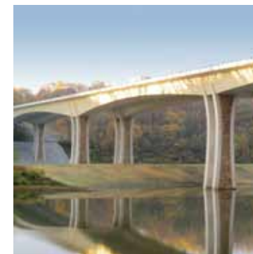
I-76 Allegheny River Bridge, PA [FIGG]
