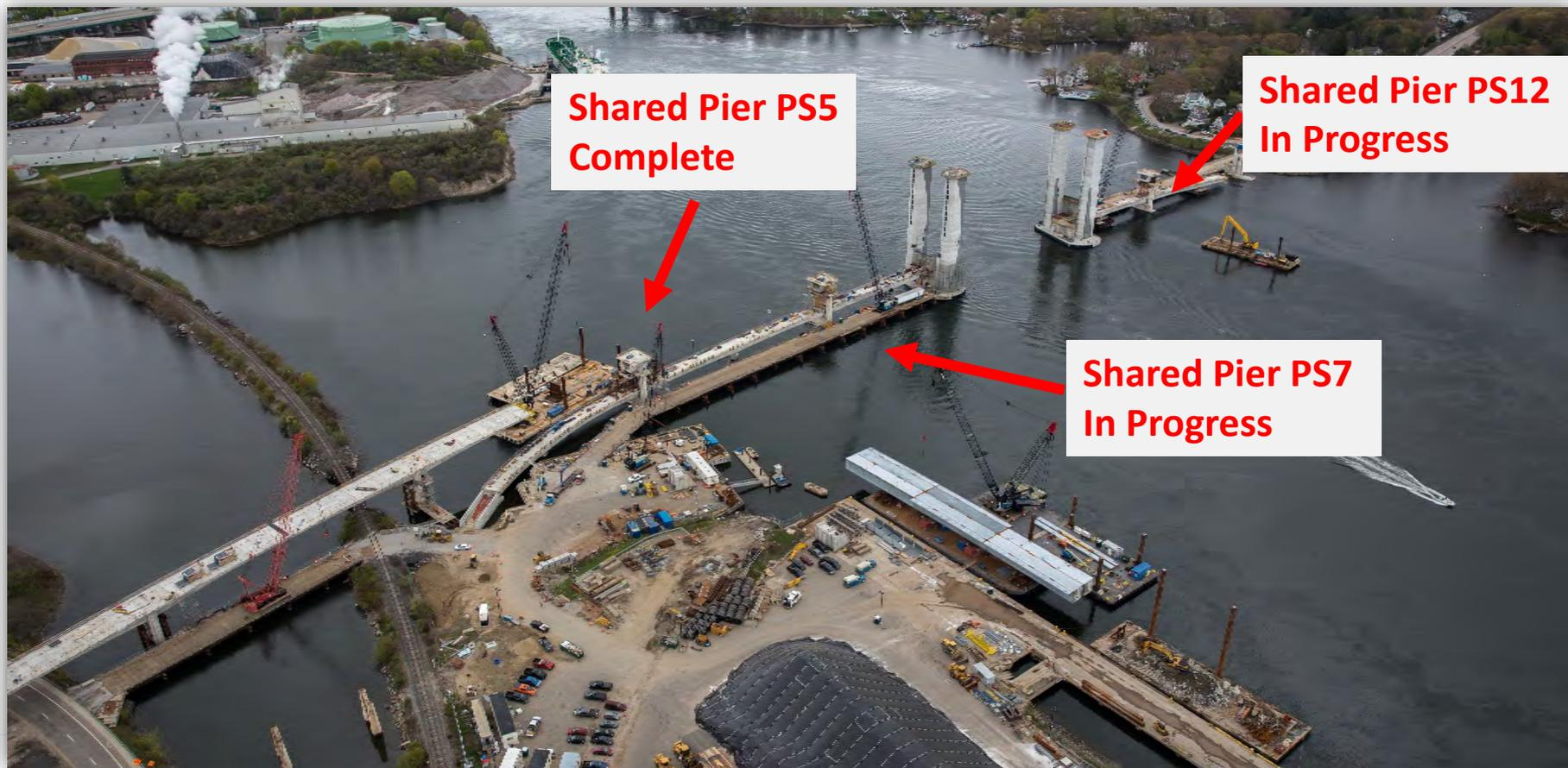
Each of the (3) shared piers are underway – segment erection has started on the PS5 cantilevers
