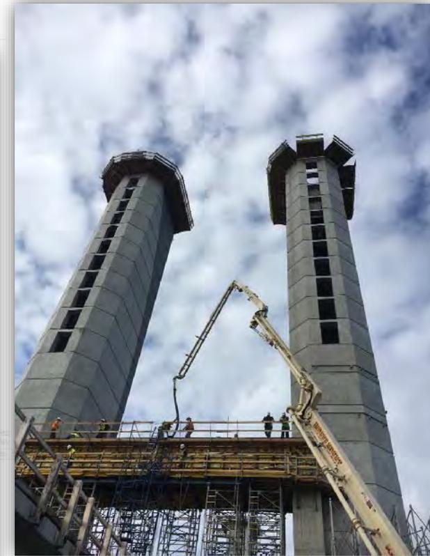
Above – Pier 9 Vehicle Approach Beam Concrete Placement
