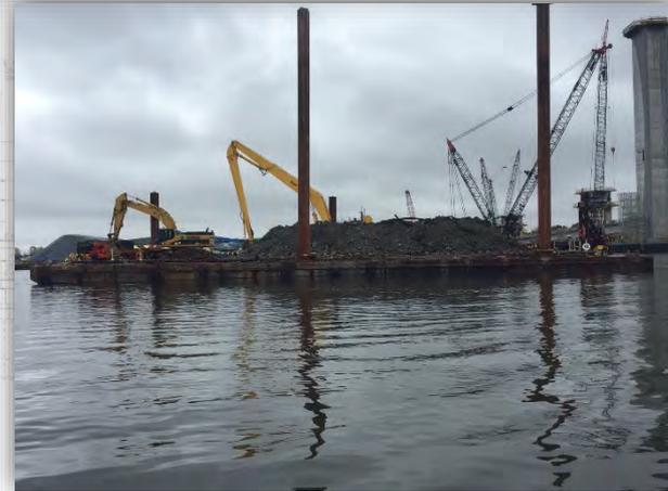
In-water piers in the main channel have been blasted. Atlantic Dismantling is currently removing demolition debris.
