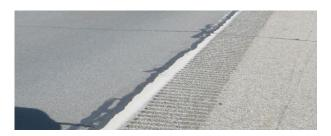
Centerline rumble strips are the most common treatment installed on Maine's two-lane roads. They are designed to alert drivers who may be heading for a potentially deadly head-on collision.
