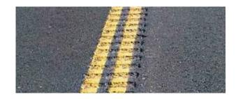
Maine rumble strips will be selectively installed on roads with speed limits of 45 mph or greater. Skips in the rumble strip pattern facilitate motorcycle lane changes.
