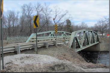
Feature on: State Route 69/220Feature under: East Branch Sebasticook RiverType: Truss (Pony)Design: Warren (Riveted)Superstructure: SteelSubstructure: ConcreteRailing type: 2 rail high steel channel;<br/>metal lattice railingNumber of Spans: 1Overall Length: 94'Deck Width: 23'Year Built: 1936Alteration (Date): n/aDesigner/Builder: MSHC/Berlin Construction Company/Edmond Cyr
