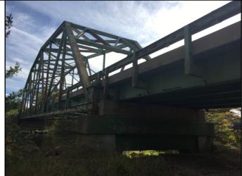
Feature on: State Route 11 Type: Truss (Thru) Superstructure: Steel Railing type: 1 high steel channel Overall Length: 369' Year Built: 1948 Designer/Builder: MSHC/American Bridge Company
