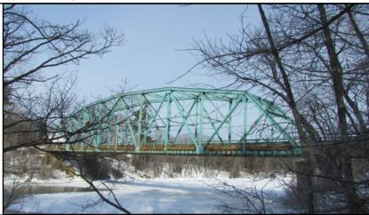
Feature on: State Route 197Feature under: Eastern RiverType: Truss (Thru)Design: Warren (Riveted)Superstructure: SteelSubstructure: ConcreteRailing type: 2 rail high steel channelNumber of Spans: 1Overall Length: 296'Deck Width: 23'Year Built: 1936Alteration (Date): n/aDesigner/Builder: MSHC & Fay, Spofford, & Thorndike/Pittsburgh-Des Moines SteelCompany/F. W. Carlton
