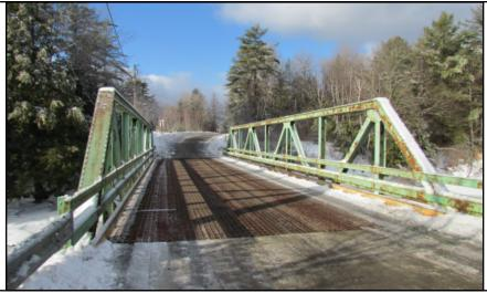
Feature on: Back RoadFeature undeType: Truss (Pony)Design: WarreSuperstructure: SteelSubstructureRailing type: 2 high steel channelNumber of SpOverall Length: 101'Deck Width:Year Built: ca. 1940Alteration (DaDesigner/Builder: MSHC/Berlin ConstructionCompany
