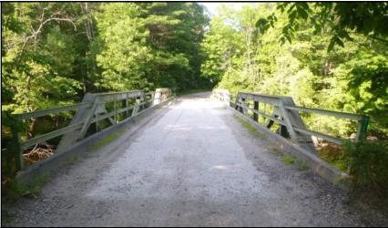
Feature on: Millturn/Salt Pond RoadFeatureType: Truss (Pony)Designerstructure: SteelSuperstructure: Steel channelNumber of the steelOverall Length: 111'Designer/Built: 1923Vear Built: 1923AlterDesigner/Builder: MSHC/United Construction Company
