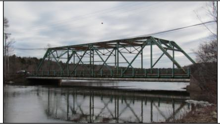
Feature on: State Route 24 Type: Truss (Thru) Superstructure: Steel Railing type: Two high steel channel Overall Length: 156' Year Built: 1953 Designer/Builder: MSCH/Herbert C. Callahan Feature under: Cathance River Design: Warren (Riveted) Substructure: Concrete Number of Spans: 1 Deck Width: 25.9' Alteration (Date): 2000
