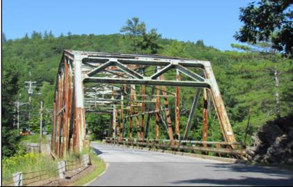
Feature on: South Rumford RoadFeature under: Androscoggin RiverType: Truss (Thru)Design: Camelback (Riveted)Superstructure: SteelSubstructure: Concrete/GraniteRailing type: 2 high steel channelNumber of Spans: 1Overall Length: 205'Deck Width: 35'Year Built: 1951Alteration (Date): n/aDesigner/Builder: MSHC/American Bridge Company
