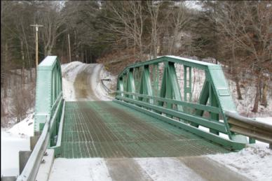
Feature on: Goulds Ridge RoadFeatType: Truss (Pony)DesSuperstructure: SteelSubRailing type: 2 high steel channelNumOverall Length: 109DecYear Built: 1937AlteDesigner/Builder: MSHC/Pan American Bridge Company
