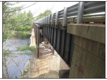
Feature on: Trestle RoadFeature under: Piscataquis RiverType: Truss (Deck)Design: Warren (Riveted)Superstructure: SteelSubstructure: ConcreteRailing type: Metal guardrailNumber of Spans: 3Overall Length: 607'Deck Width: 15'Year Built: 1947Alteration (Date): 1981Designer/Builder: Bangor & Aroostook Railroad/Bethlehem Steel Company
