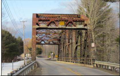
Feature on: State Route 106Feature under: Dead RiverType: Truss (Thru)Design: Pennsylvania (Riveted)Superstructure: SteelSubstructure: ConcreteRailing type: 2 high steel channelNumber of Spans: 1Overall Length: 177'Deck Width: 21'Year Built: 1922Alteration (Date): 1974, 1988Designer/Builder: MSHC Bridge Division/United Construction Company
