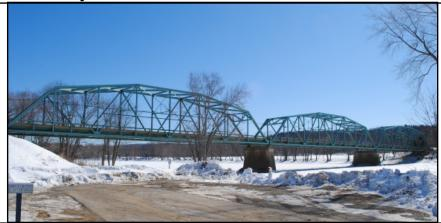
Feature on: Chester RoadFeature under: Penobscot RiverType: Truss (Thru)Design: Warren (Riveted)Superstructure: SteelSubstructure: ConcreteRailing type: 1 high steel channelNumber of Spans: 3Overall Length: 610'Deck Width: 23.6Year Built: 1950Alteration (Date): 1983Designer/Builder: MSHC/Lackawanna Steel Construction Corporation
