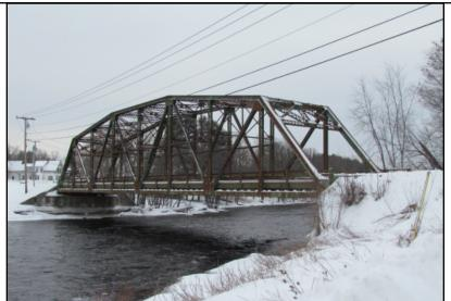
Feature on: Pleasant StreetFeature under: Sebasticook RiverType: Truss (Thru)Design: Warren (Riveted)Superstructure: SteelSubstructure: ConcreteRailing type: 2 rail high steel channel;<br/>metal pipe on sidewalkNumber of Spans: 1Overall Length: 190'Deck Width: 23'Year Built: 1936Alteration (Date): n/aDesigner/Builder: MSHC/American Bridge Company/J. R. Cianchette & Company
