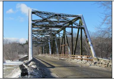
Feature on: Pleasant StreetFeature under: Pleasant RiverType: Truss (Thru)Design: Warren (Riveted)Superstructure: SteelSubstructure: ConcreteRailing type: 2 rail high steel channelNumber of Spans: 2Overall Length: 309'Deck Width: 23'Year Built: 1936Alteration (Date): n/aDesigner/Builder: MSHC/Harris Structural Steel Company/W. H. McPherson
