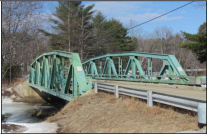
Feature on: State Park RoadFeatType: Truss (Pony)DesiSuperstructure: 2 high steel channelSubsRailing type: SteelNumOverall Length: 123'DeciYear Built: 1937AlterDesigner/Builder: MSHC/Lackawanna Steel Construction
