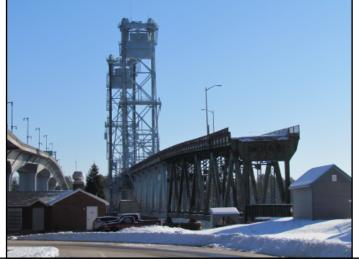
Feature on: Rockland Branch RailroadFeature under: Kennebec RiverType: Truss (Deck) & Lift SpanDesign: Warren (Riveted)Superstructure: SteelSubstructure: ConcreteRailing type: Tubular metal pipeNumber of Spans: 7with metal bar fillDeck Width: 35'Overall Length: 2,195'Deck Width: 35'Year Built: 1926-1927Alteration (Date): 2000Designer/Builder: J. A. L. Waddell/McClintic-Marshall/Foundation Company
