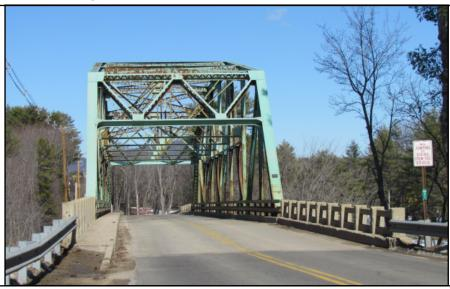
Feature on: State Route 160Feature under: Saco RiverType: Truss (Thru)Design: Warren (Riveted)Superstructure: SteelSubstructure: ConcreteRailing type: 2 rail high steel channelNumber of Spans: 1Overall Length: 339'Deck Width: 26'Year Built: 1936Alteration (Date): n/aDesigner/Builder: MSHC/Harris Structural Steel Company/Wyman & Simpson, Inc.
