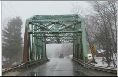
Feature on: State Route 156Feature under: Wilson StreamType: Truss (Thru)Design: Camelback (Riveted)Superstructure: SteelSubstructure: ConcreteRailing type: 2 rail high steel channelNumber of Spans: 1Overall Length: 176'Deck Width: 23'Year Built: 1937Alteration (Date): n/aDesigner/Builder: MSHC/Pittsburgh-Des Moines Steel Company/Reed & Reed
