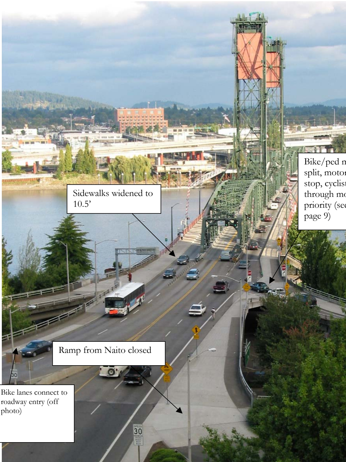
Hawthorne Bridge westside, eastbound, after improvements made.
