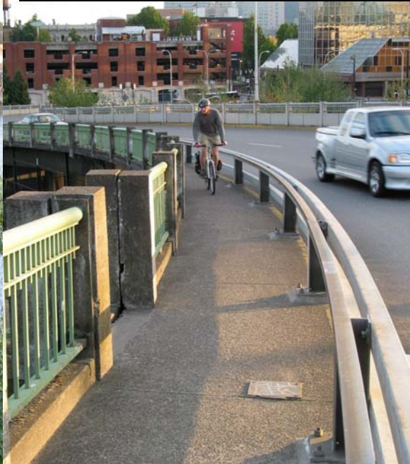
Before: Steel Bridge, upper deck. Bicyclists and pedestrians sharing one 5' sidewalk with guardrail.
