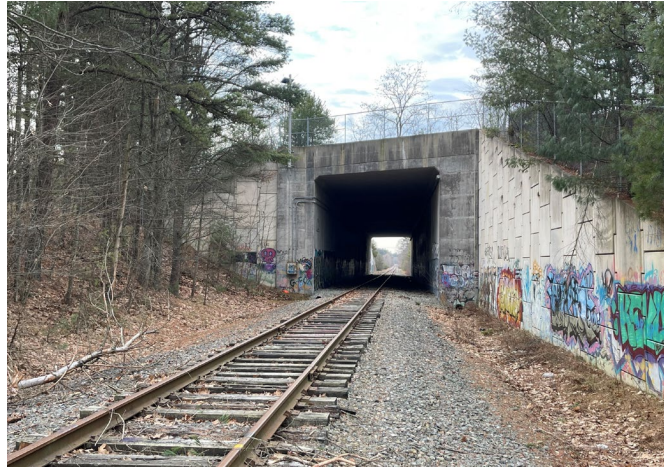
Middlesex Rd. overpass in Topsham at MP 30.54
