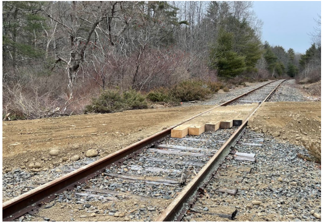
Recently replaced timber farm crossing in Richmond at MP 47.50
