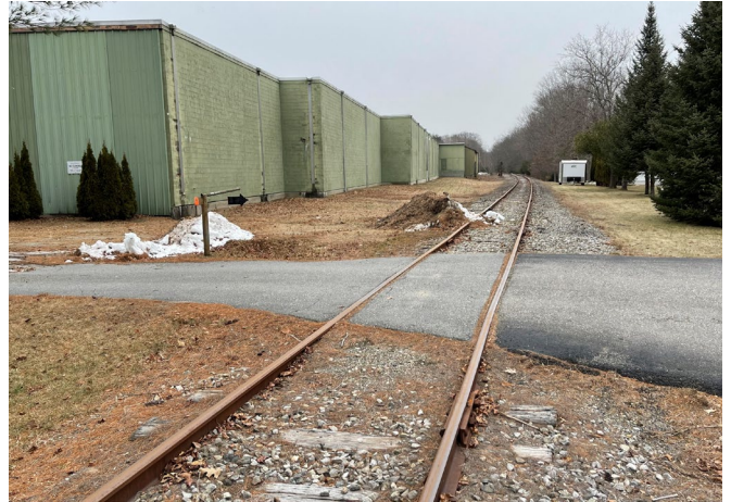
Location in Gardiner (MP 52.70) where space for a passing siding is available for potential future passenger rail service.
