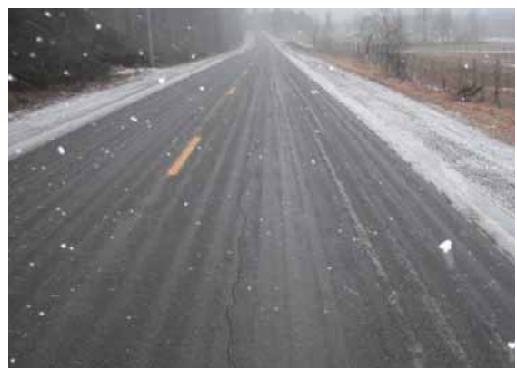
Clean road in Pownal after liquid brine application
