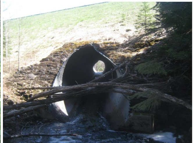
Route 1 Bridge #6248 Existing Prestile Brook Culvert
