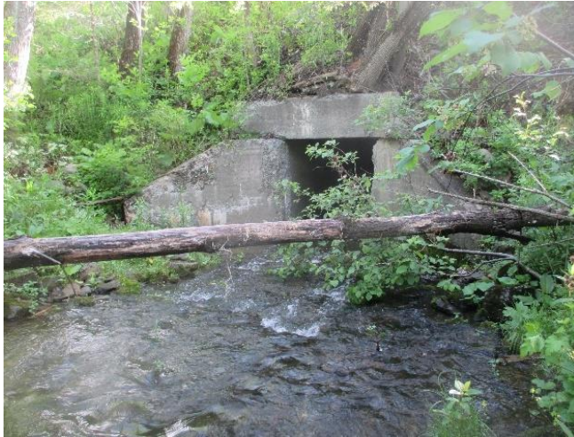
Figure 1: Route 164 Large Culvert #931080 Existing Prestile Brook Culvert
