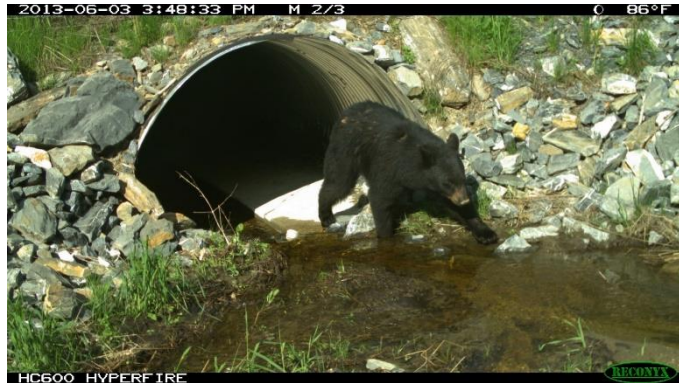
Figure 11: Caribou Bypass Culvert Wildlife Crossing source: MaineDOT
