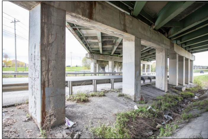
Figure 11 Under the overpass showing spalling and deterioration to the concrete.
