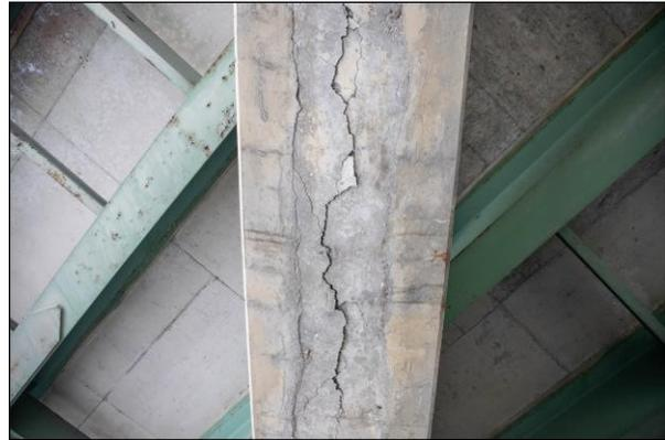
Figure 14 Cracks in concrete caps.
