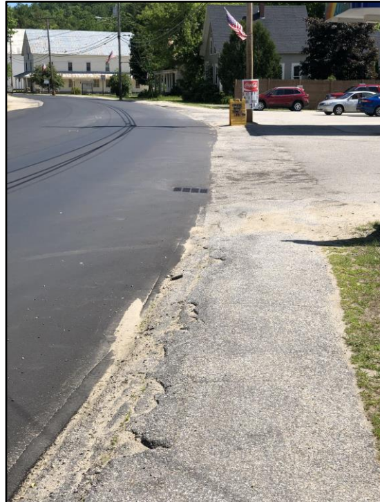
While Route 26 through Woodstock (Bryant Pond Village) recently received an asphalt topcoat, heavy truck traffic continues to weaken the old road structure underneath. A lack of bike lanes and defined sidewalks creates a safety concern for pedestrians.
