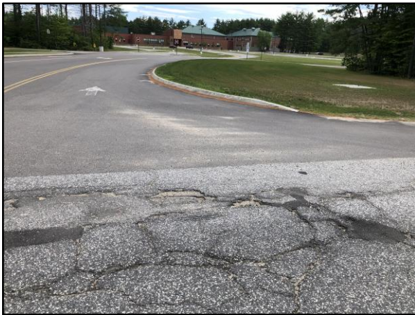
Potholes and rutting characterize the road surface of U.S. Route 302. Shown in Fryeburg in front of Molly Ockett Middle School.
