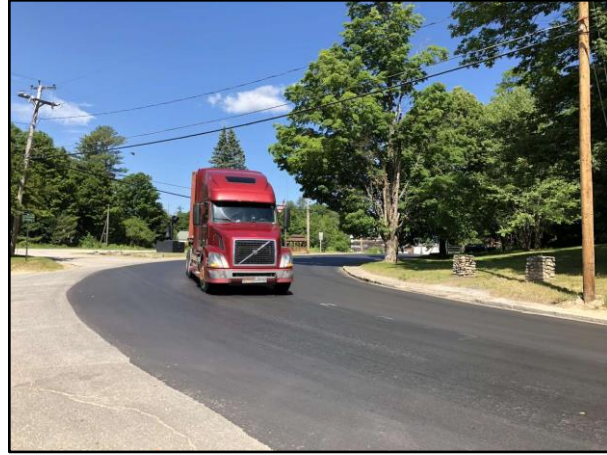
A semi-truck rounds the sharp curve in Bryant Pond Village, part of the Woodstock portion of the Project.
