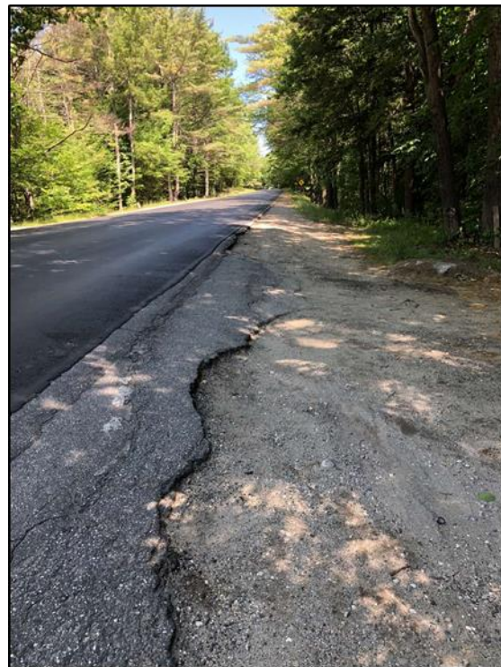
The road's current shoulder, a mix of gravel and old pavement, is a danger to bicyclists.
