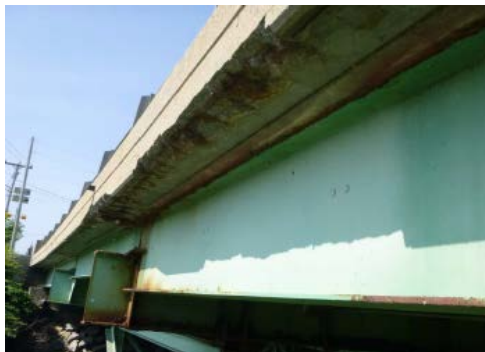
Spalled and delaminated soffit, South side
