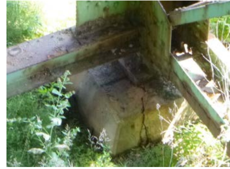
Cracking of the center column, 6th bent
