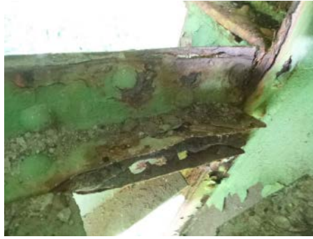
Section loss on bracing
