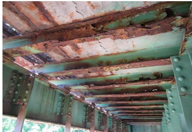
**Figure 8: Deteriorated crossbeams & deck**
