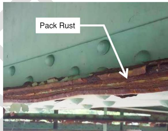
**Figure 17: Pack rust is corrosion in the crevice between two plates of steel that are bolted or riveted together. As the rust progresses, it gradually pushes the pieces of steel apart, bending them and sometimes breaking bolts or rivets. To truly fix pack rust, the members need to be taken apart and thoroughly cleaned, which is a complex and expensive effort.**
