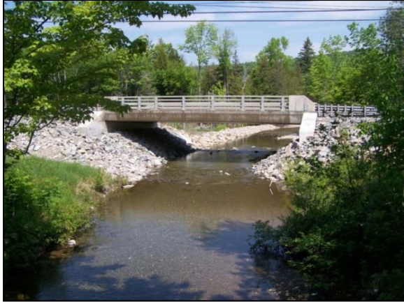
Single span bridge (40' to 60')
