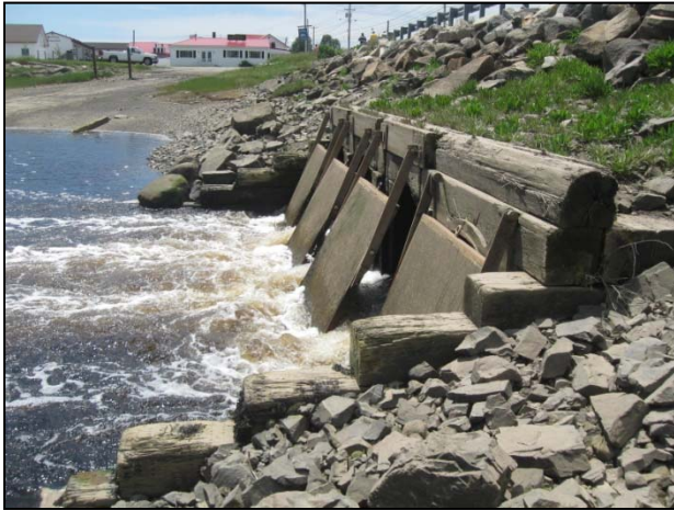
Existing Dyke Bridge Structure
