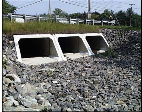
Multiple adjacent culverts
