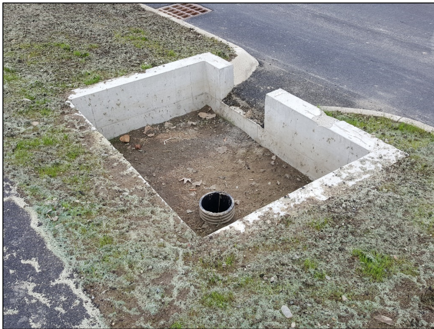
Construction of a stormwater planter in Orono, ME.
