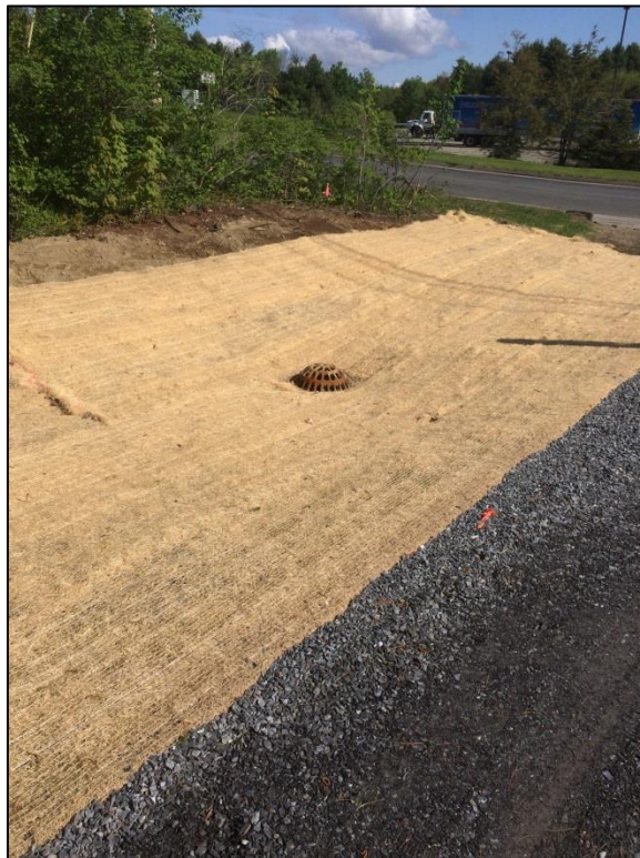
Underdrained filter ditch.
