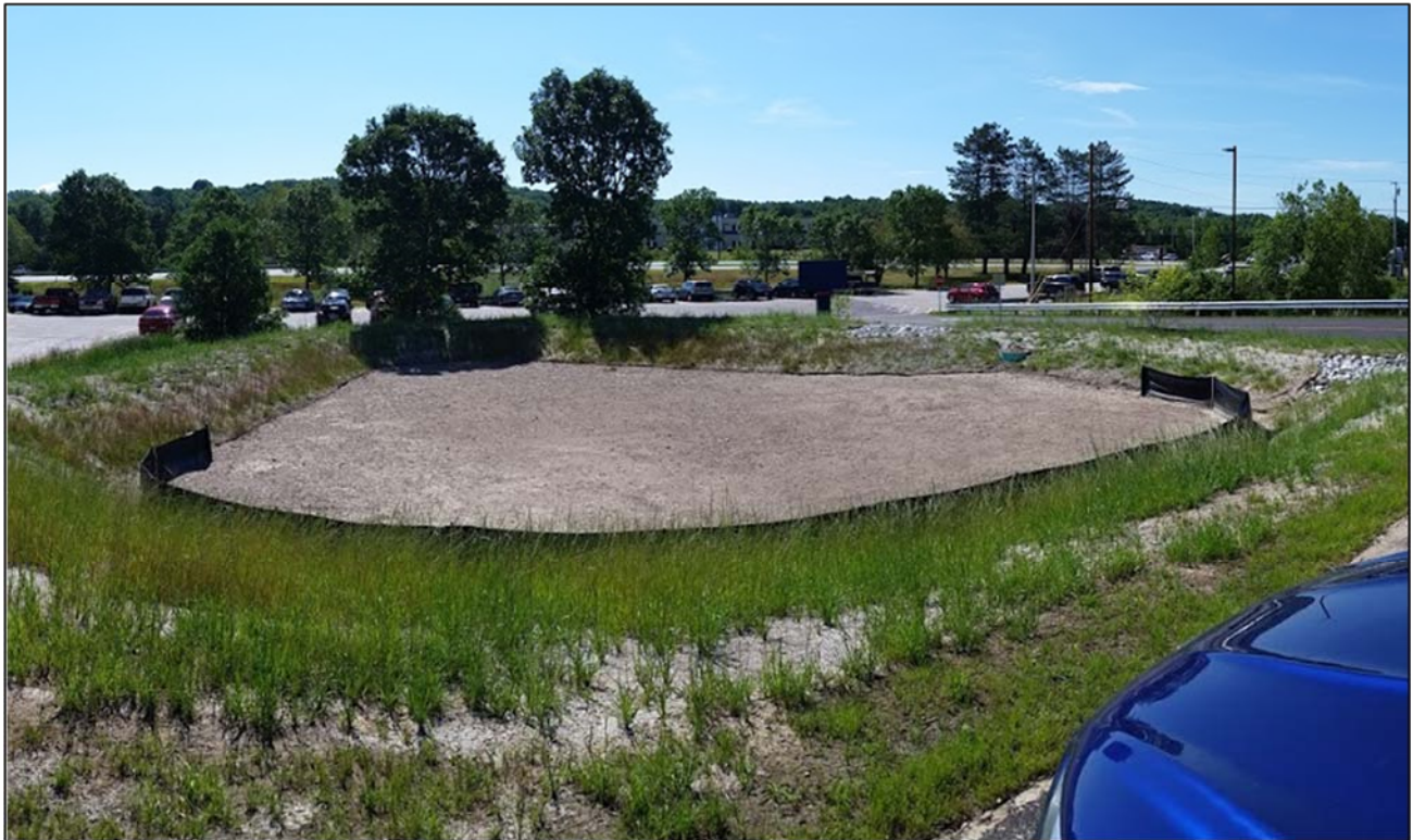
Constructing a Stormwater Infiltration Basin for the Auburn Bus Station project, 2017.
