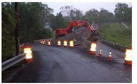
On June 16th, a teenager walking along Route 24 in Harpswell fell into a sinkhole adjacent to the road. Further investigation revealed that a 30-inch diameter, 106- foot long metal cross culvert had corroded and failed. By nightfall, a MaineDOT crew had filled the hole and barricaded the site. Plans were devised to immediately replace the pipe. The project was complex, since the pipe was 24 feet below the
