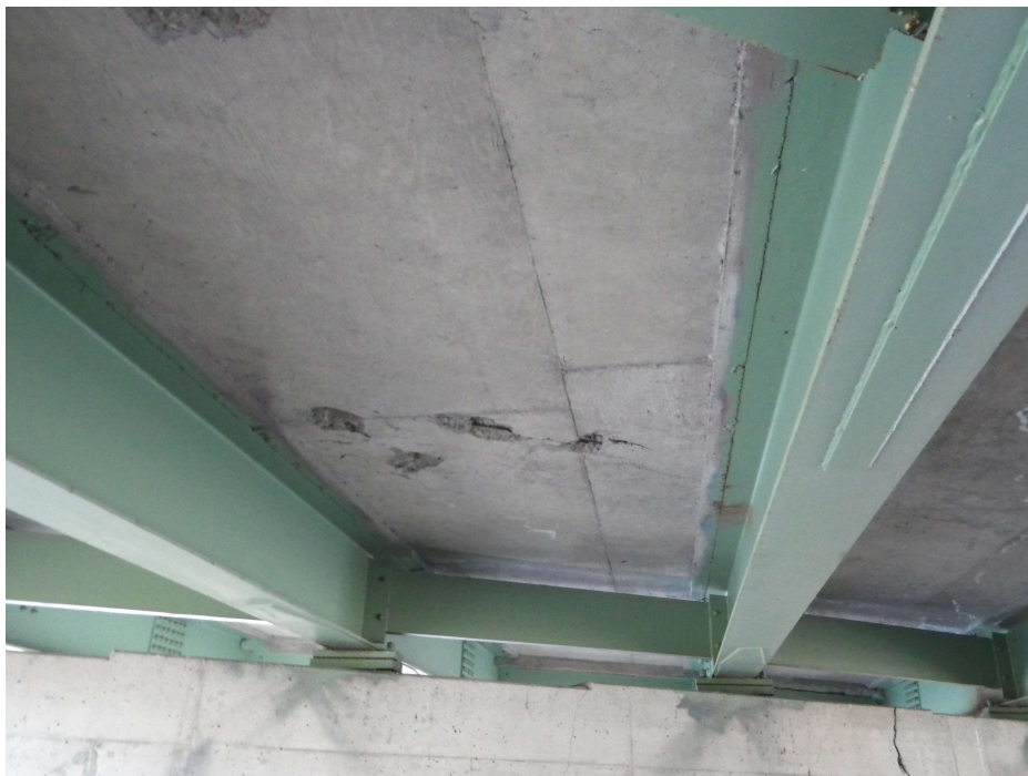
PHOTO 8 Description Spalled areas on bottom of deck, West end
