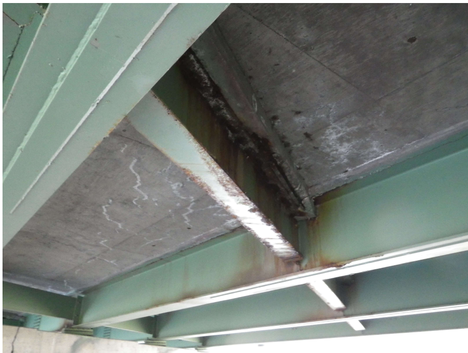
PHOTO 7 Condition Description Leaking deck with steel deterioration below
