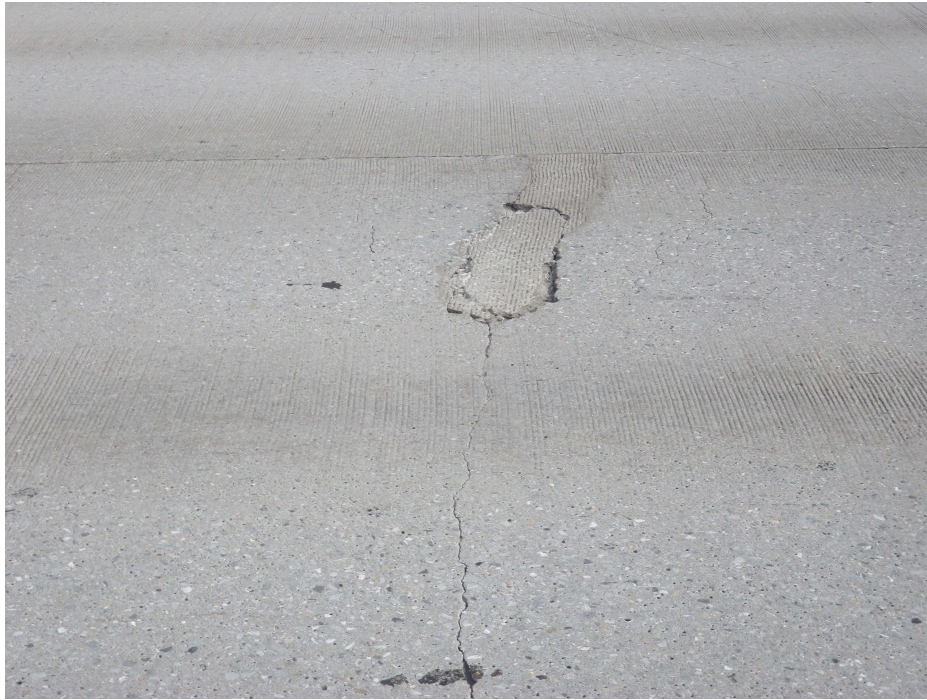
PHOTO 17 Condition Description Area of delaminated concrete in wearing surface
