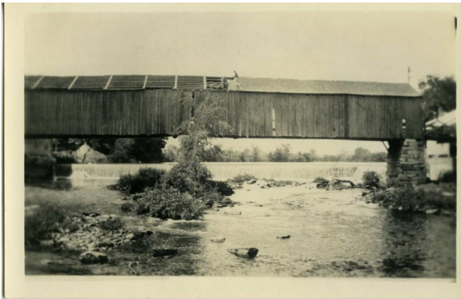
Figure 1- Looking upstream at covered bridge pre 1931. Image courtesy of the Farmington Historical Society.
