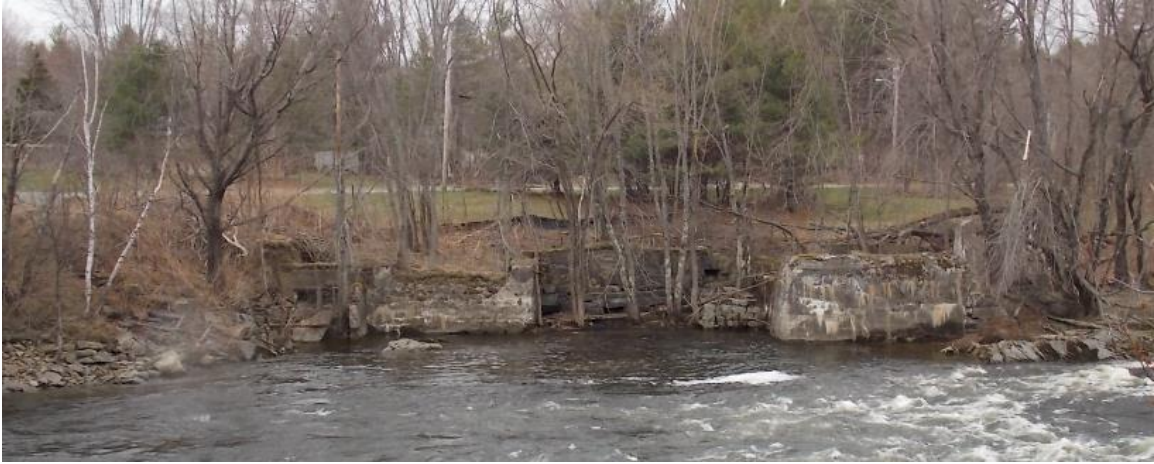
Figure 11- Looking southwest from existing bridge at the remains of old foundations
