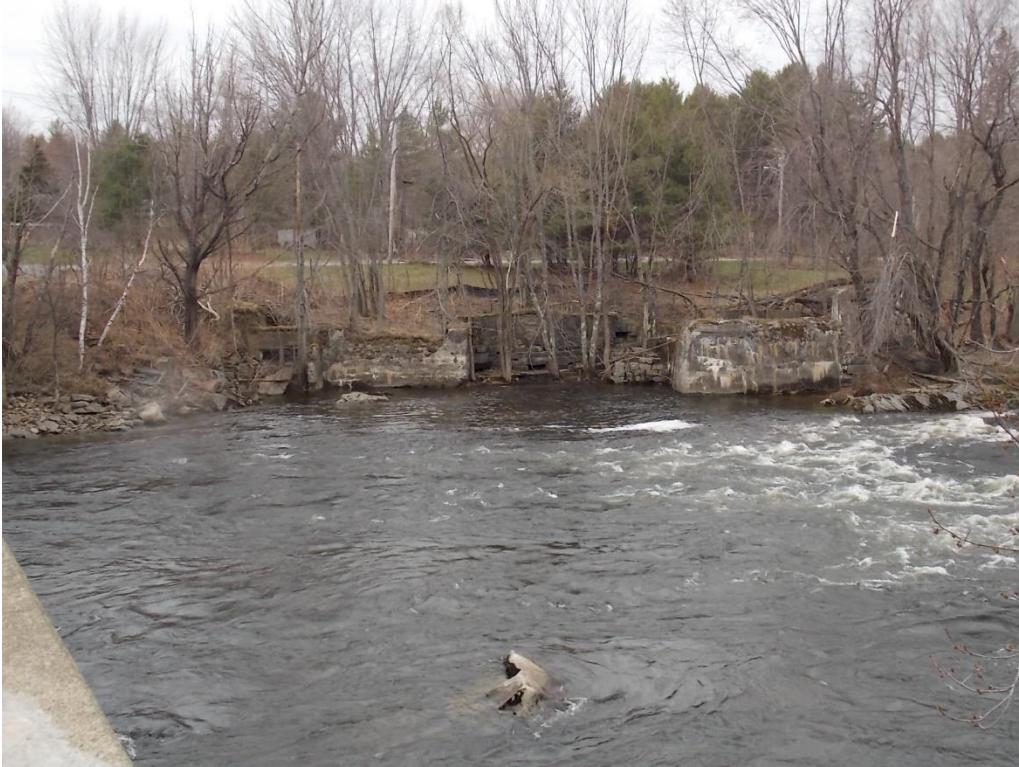
Old foundations southwest of the existing bridge
