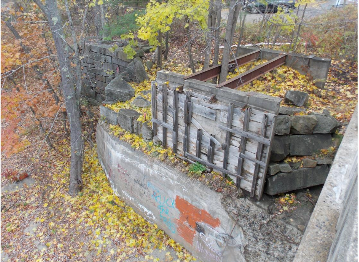
Figure 7 - Old foundations located at the northwest corner of the existing bridge
