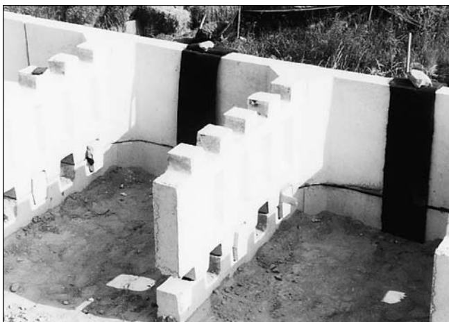
Filter fabric covering vertical joints on back face
