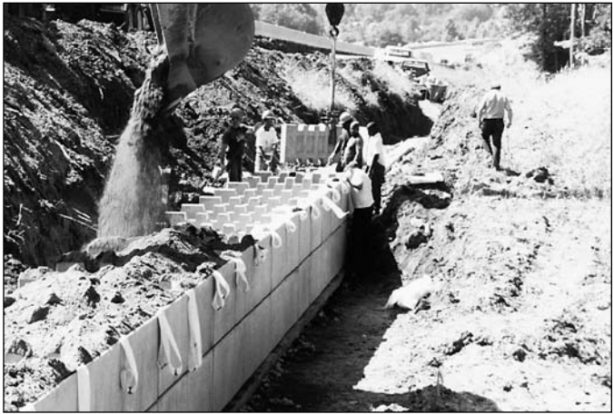
Placing the backfill
