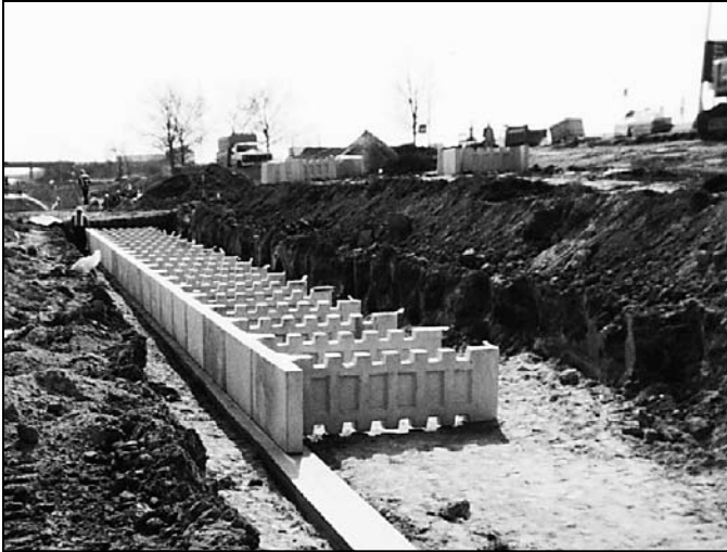
First course of units on leveling pad
