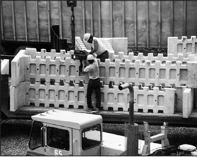
Unloading units from truck
