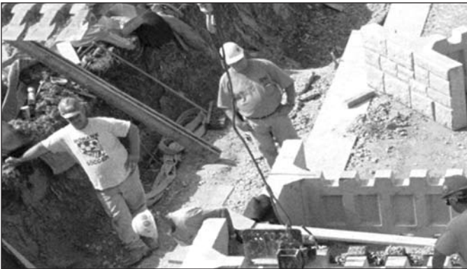
Rigging and setting a T-WALL® unit
