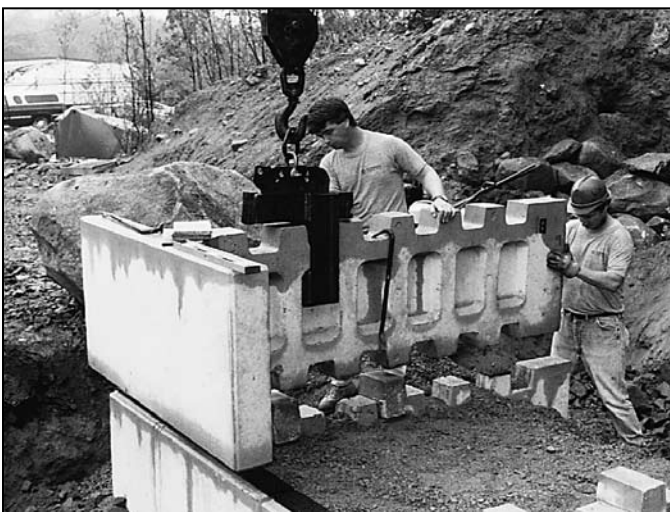
Putting units into position
