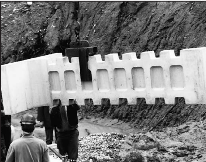
Lifting a 10' unit at the balance point
