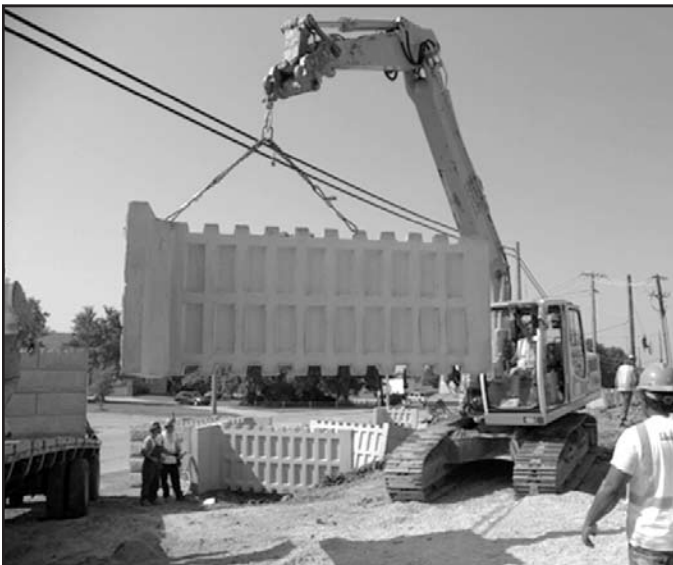
Lifting a double unit which was precast with lifting inserts
