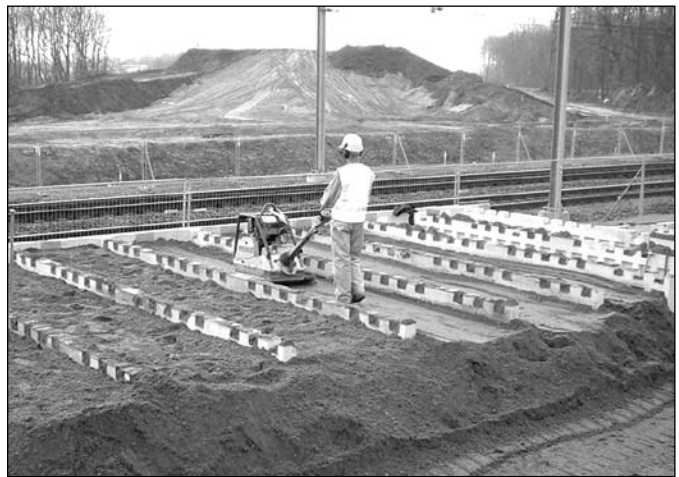
Compacting the backfill
