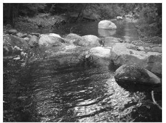
Figure 10. Rock weir with embedded root wad constructed in 2007 showing scoured pool. Sandy River, Maine. Photo credit F. Bonney.
