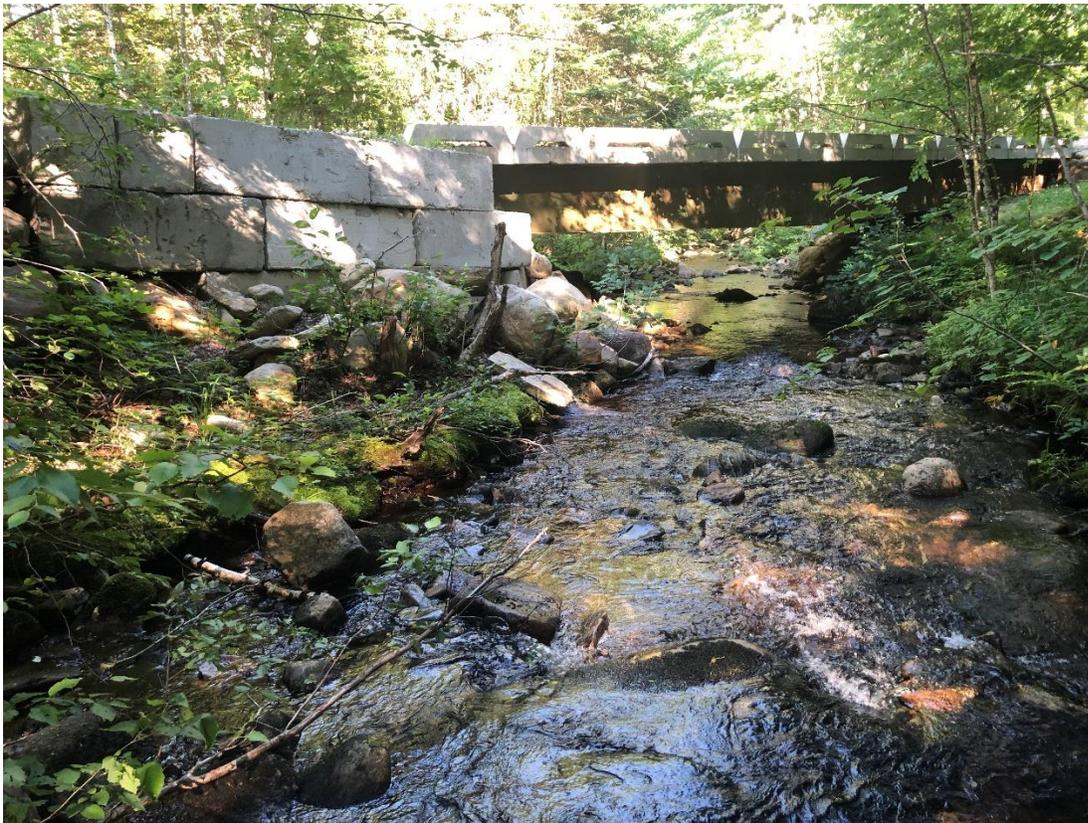
This crossing is constructed with commercially available modular concrete blocks. It is greater than full bank width and retains the natural substrate. Photo by Chuck Hulse, MDIFW
