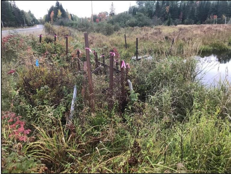
This enclosure has been working for 30 years despite the fencing having long since deteriorated. This is because beaver constructed a dam against the fence when it was installed. The culvert opening is clear and out of view, 20 feet left of the fence.
