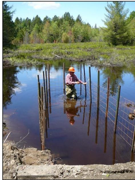
Beaver are hard-wired to build *perpendicular* to the waterflow, so having a large percentage of the enclosure perimeter aligned parallel to the water course is meant to “deceive” them. This design was developed by wildlife biologist Skip Lyle.
