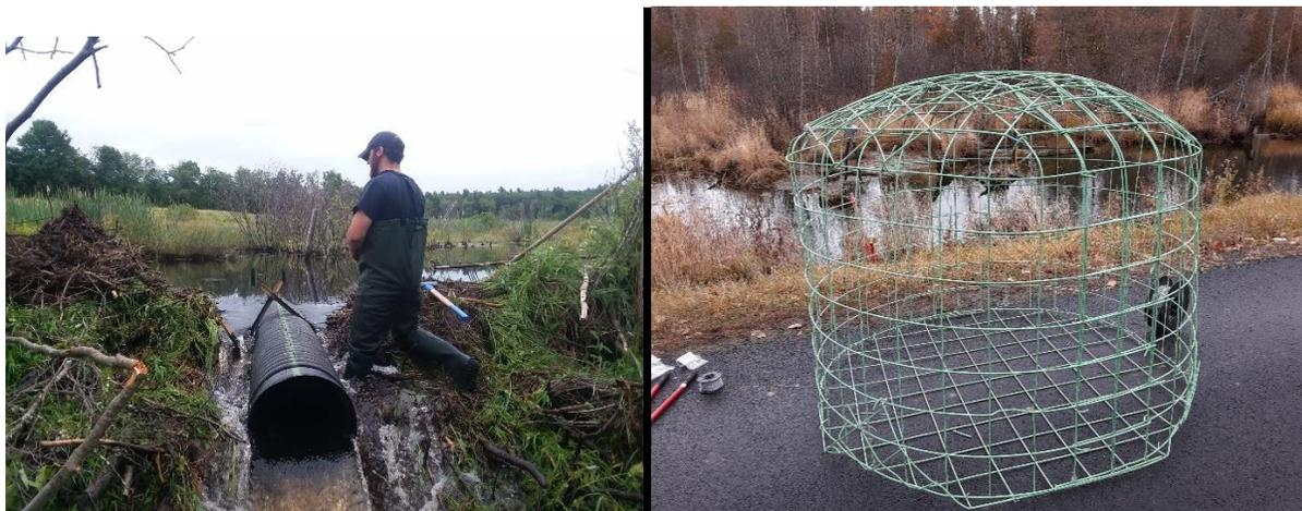
The upstream end of the leveler can be placed in a sunken cage made from livestock panel fencing. To extend the life of the cage, use epoxy coated wire mesh as shown in the right image. If holes are drilled in the water leveler it does not to be level. Tip: The farther the cage is from the dam the harder it is for beaver to determine the origin of the leak. With a plastic culvert use a minimum of one 20-footer. Photos by Ben Nugent, USDA-Wildlife Services
