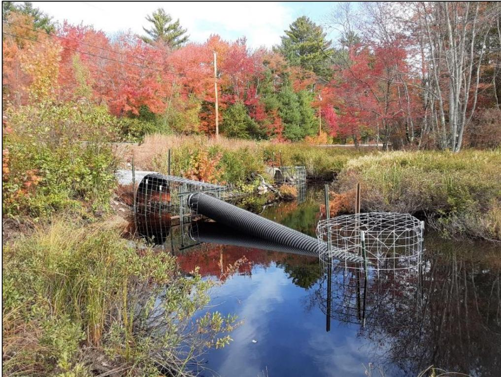
Exclosures are constructed with livestock panel fencing. Both were built on dry ground nearby. The white-tipped T-Posts were put in place with a light, hand-held fencepost pounder. Photo by Chuck Hulsey, MDIFW
