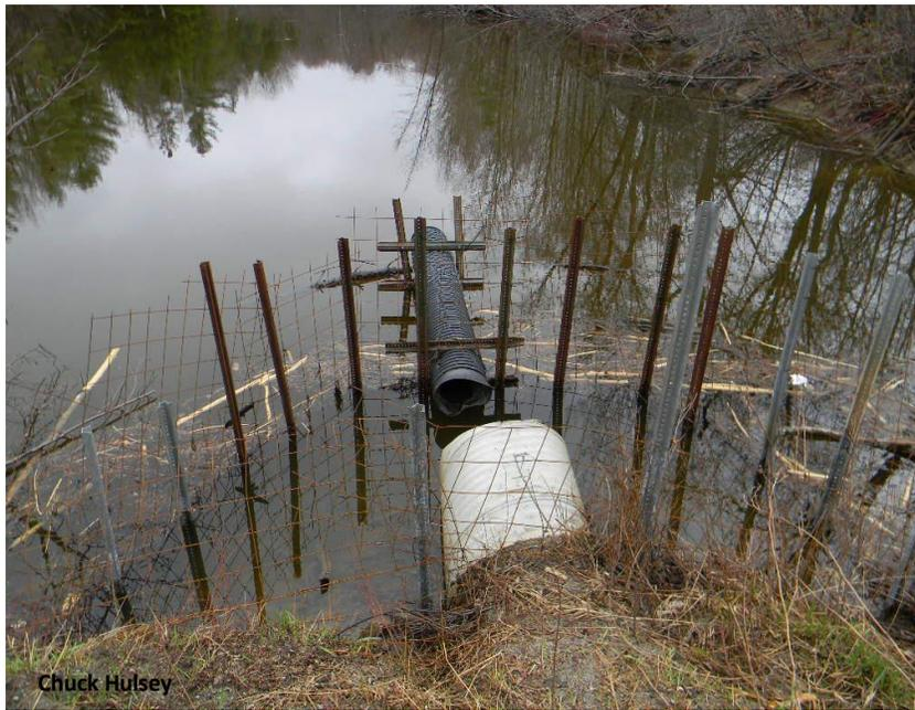
Arc-shape enclosure with channel post and concrete reinforcement wire. The leveler is made from a piece of salvage plastic culvert, with the end blocked and a slot on the underside to receive water. **NOTE:** Leave a gap on one side, between the first post and the shore if turtle passage is a concern.
