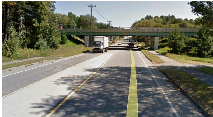
Figure 77: Looking South along 302 at I-95 overpass
