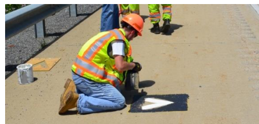
Figure 79: Typical Target installation
