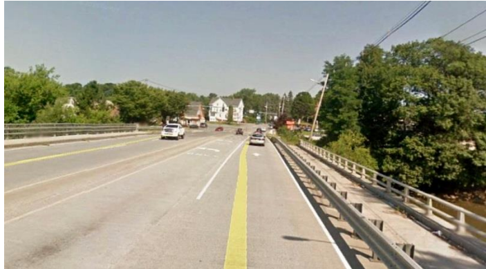
Figure 78: Looking North along 302 at Bridge over Presumpscot River
