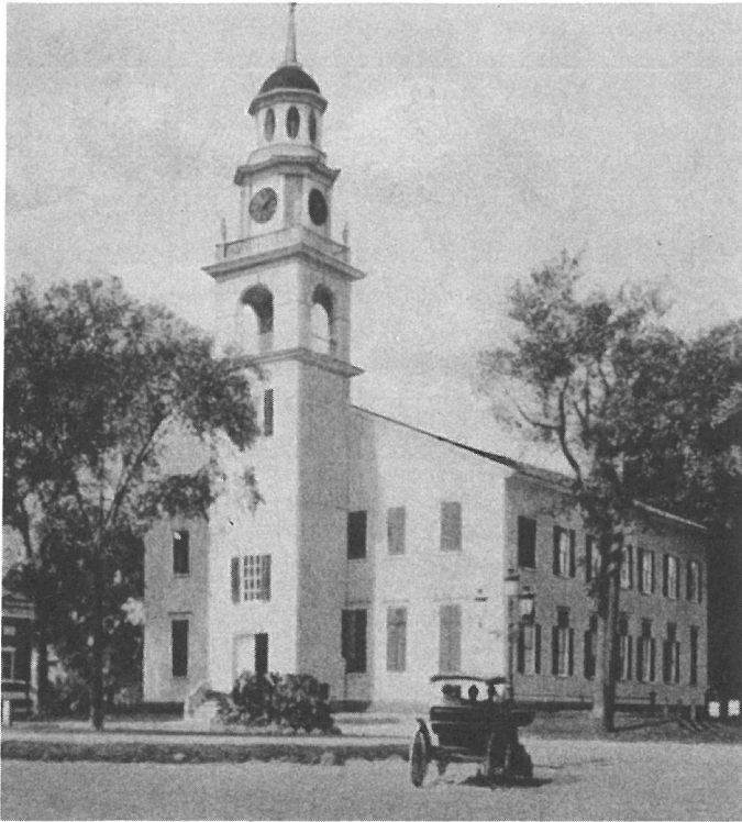
Figure 3. First Parish Church, Kennebunk, 1909 view (MHPC).
