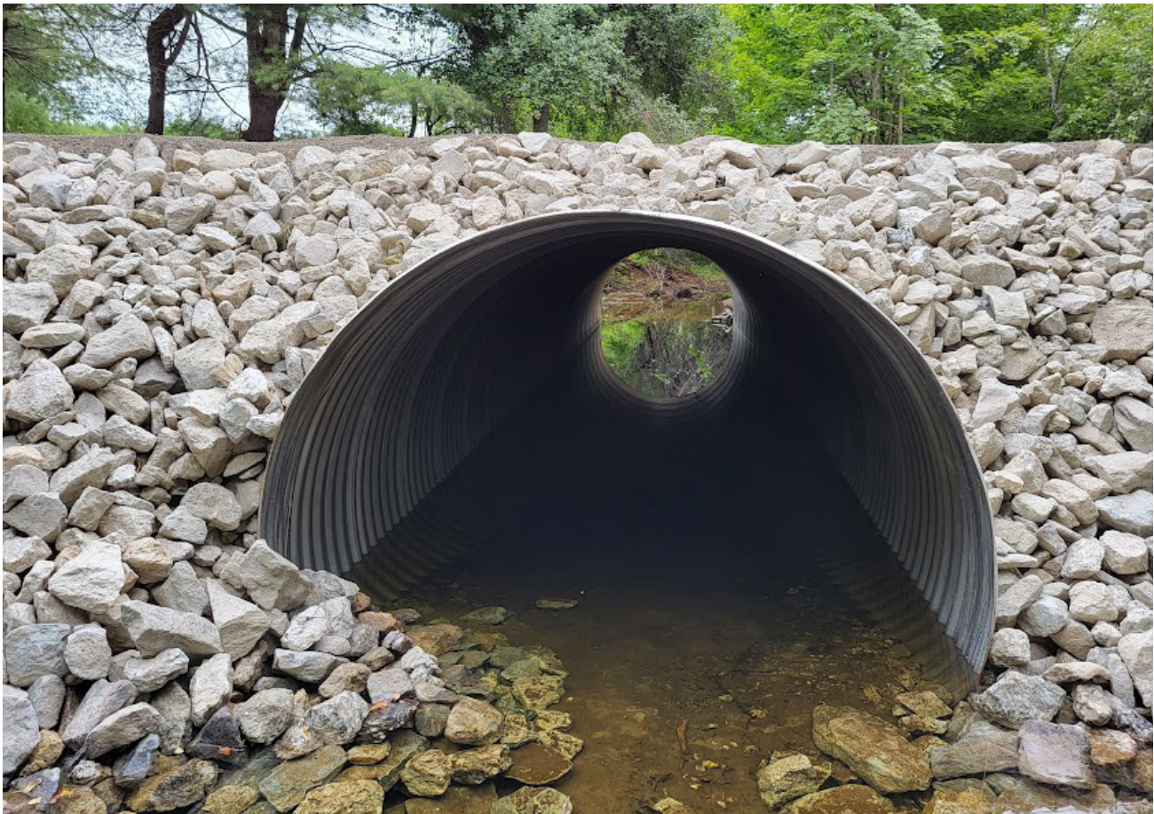
This culvert in Paris, Maine was constructed in 2023 to withstand extreme weather events, and was undamaged during the storms in 2024. Credit: Maine DOT
