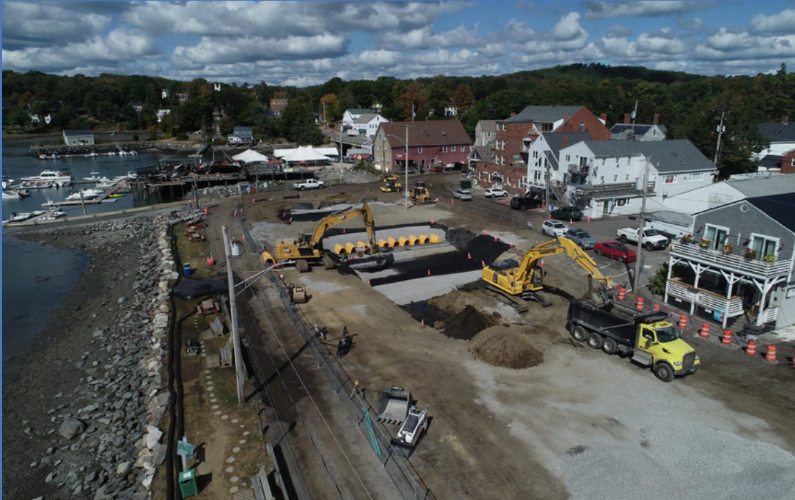
A work crew wraps up installation of the new underground stormwater retention system in Damariscotta last September. Credit: Town of Damariscotta
