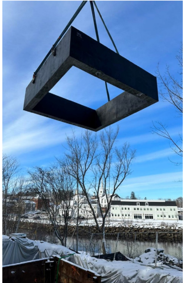
Part of the well for the Southside Pump Station in Machias is installed in 2023. The pump station was part of a 10 year upgrade to reduce overflow events at the Machias Wastewater Treatment Plant. Credit: Town of Machias
