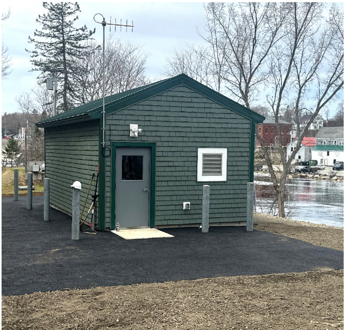
Now completed, the new pump station is located on higher ground, above the flood line on the south side of the Machias River in Machias. Credit: Town of Machias
