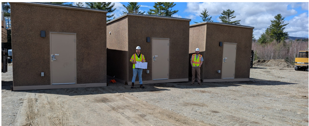
Precast colocation huts, which weigh around 63,000 lbs each, were delivered to the Central Maine Crane Yard in Avon in April. Built with reinforced concrete, integrated electrical, HVAC, and grounding systems, these heavy-duty structures will eventually be installed at their final locations by Sertex Broadband Solutions to complete the MOOSE NET Middle Mile Program’s plans to expand broadband access across Maine. Credit: Maine Connectivity Authority
