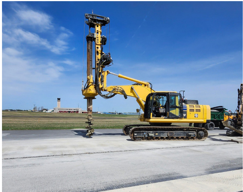
Projects include runway improvements and terminal upgrades — including the connector bridge (cover photo), which links the domestic and international terminals post-security at Bangor International Airport. Credit: Bangor International Airport.
