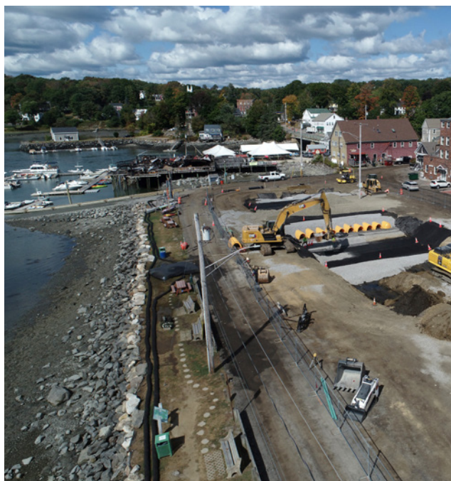
In September 2024, work crews completed installation of the new large-scale underground stormwater retention system to help prevent coastal flooding in Damariscotta. Credit: Town of Damariscotta
