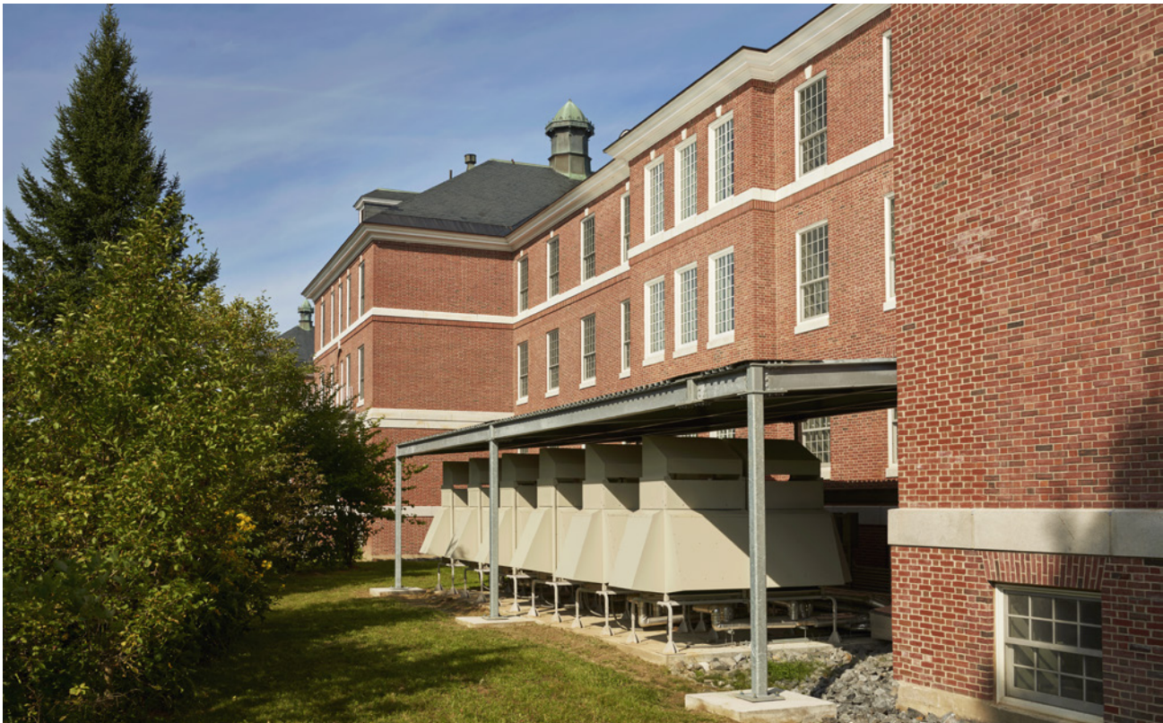
Air cooled variable refrigerant flow high efficiency heat pumps in the Ray building in Augusta. Photo credit: Darren Setlow
