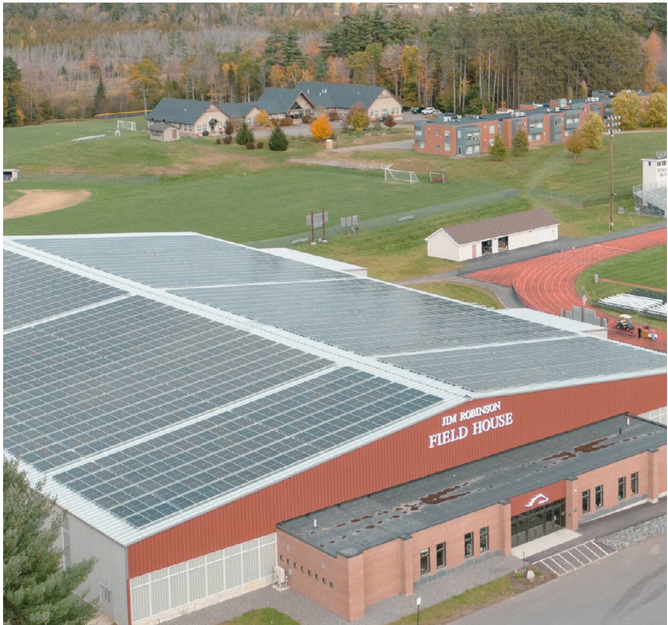
A 1-megawatt community solar farm was installed on the roof of the field house at Foxcroft Academy. This farm, which offsets over 1,200 metric tons of carbon dioxide annually, provides energy for Foxcroft Academy and the local public school district, RSU 68. Approximately 500 students, educators, community members, and government officials attended the project's celebration event. Photo Credit: Foxcroft Academy
