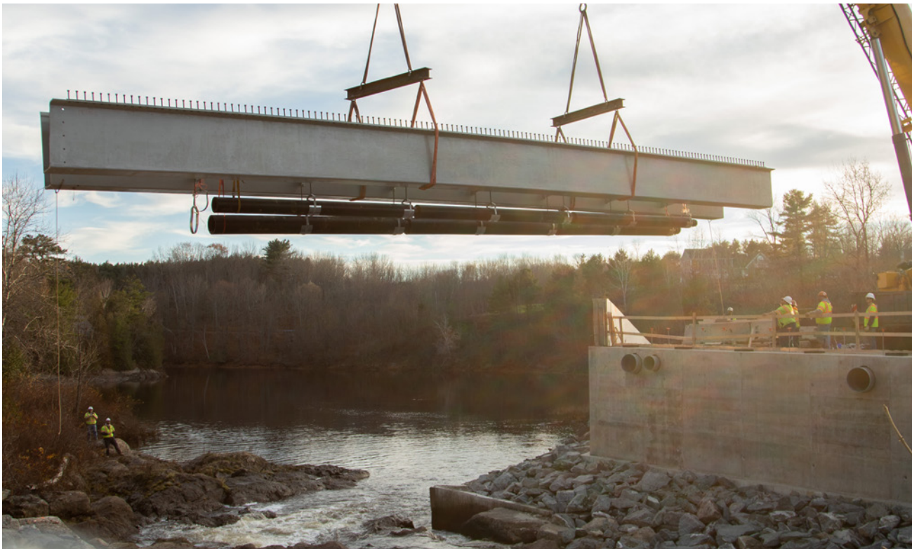
Construction of the Grist Mill Bridge in Hampden. The new bridge is the first in the nation to use fiber-reinforced polymer tub girders called GBeams, a patented technology resulting from research and development at the UMaine Composites Center. Photo credit: Maine Department of Transportation.
