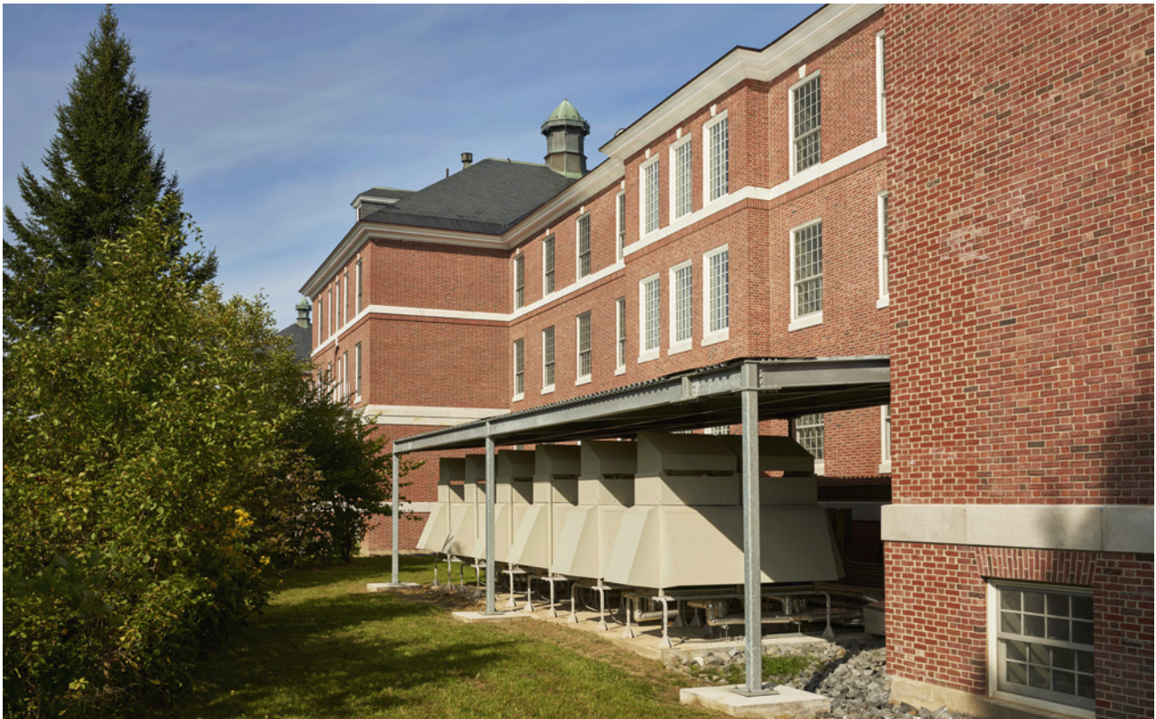
Air cooled variable refrigerant flow high efficiency heat pumps in the Ray building in Augusta. Photo credit: Darren Setlow
