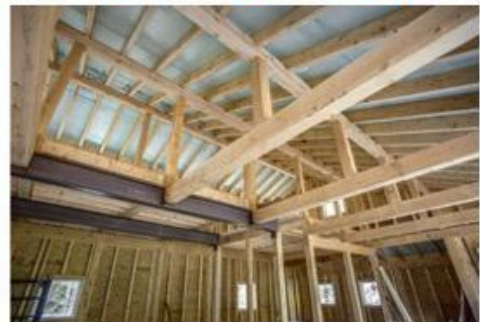
Interior of an efficient post and beam home, constructed by Burnham & Lebowitz Builders in Freeport. It was constructed using a continuous, air-tight, well-insulated exterior outer shell with R-35 walls and an R-65 roof. Photo by Tim Greenway.
