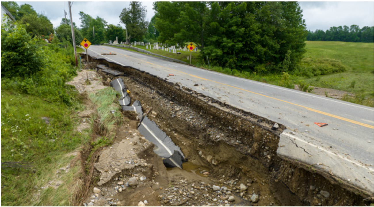
Parts of Route 133 in Jay, Maine sustained heavy damage from runoff during an historic summer rainfall in June 2023 that required months of repairs.
