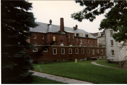
The Central Building with 1958 1 st floor addition.
