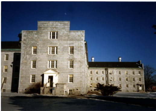
Stone South and Southeast.
