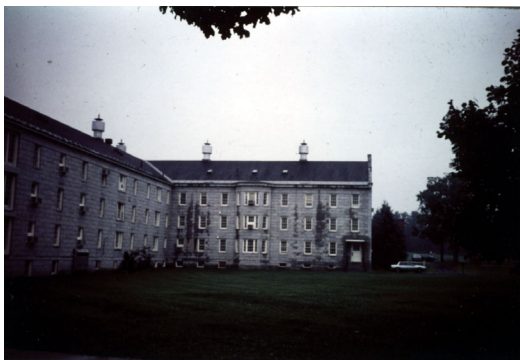
Roof ventilators such as these on the roof of Stone South were important parts of the original building ventilation systems.
