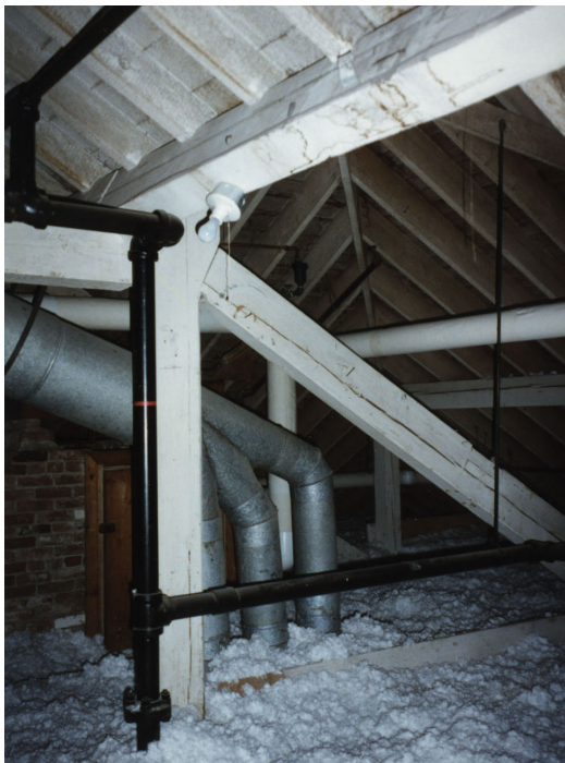
The roof structures of all the Stone Complex buildings are similar.
