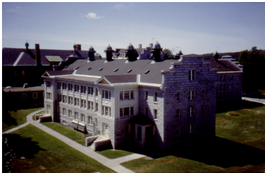
Most AMHI buildings such as Stone North, will lend themselves graciously to new office use.
