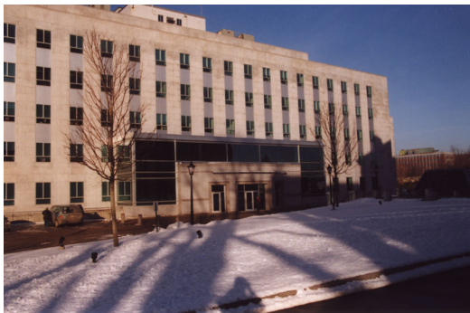
The newly renovated Burton M. Cross State Office Building.
