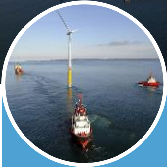
Navigation Channel and Wet Storage
