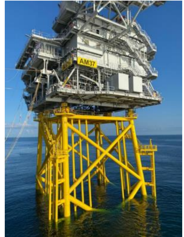
Vineyard Wind 1 Substation Photo Courtesy of Vineyard Wind
