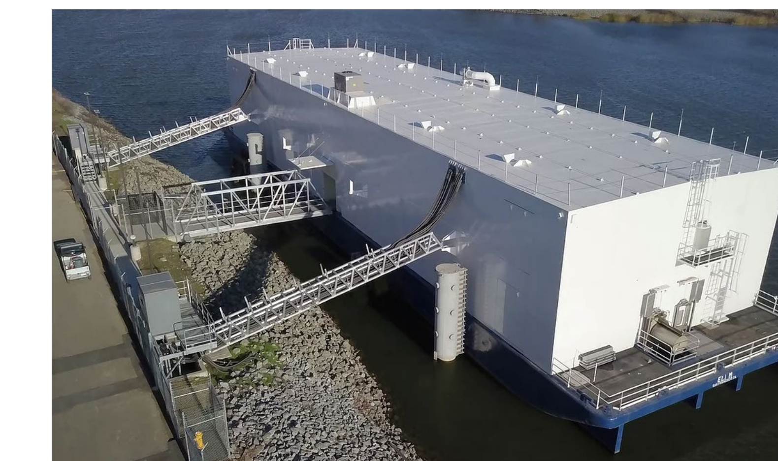
Fig. 12: Nautilus Data Technologies' Stockton1 facility, CA. Source: Nautilus (2021) . [Saline/Non-potable water cooling]
