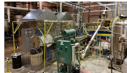
0.1 tpd Synthetic Crude Oil Pilot Plant (SynCOPP)
