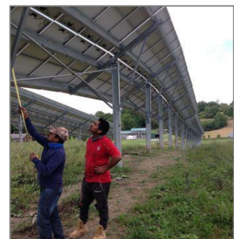
Figure 7: Raised Array at Maple Ridge Meats. Source: ruralsolarstories.org
