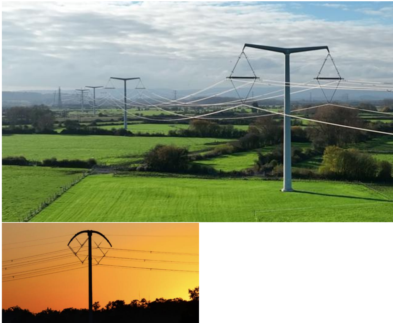
Figure 27: (Left) T-Pylon structures 133 ; (Right) Curved steel structures 134
