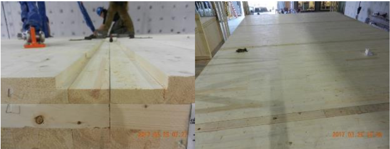
Figure 7. Ceiling panels connected with spline joints.
