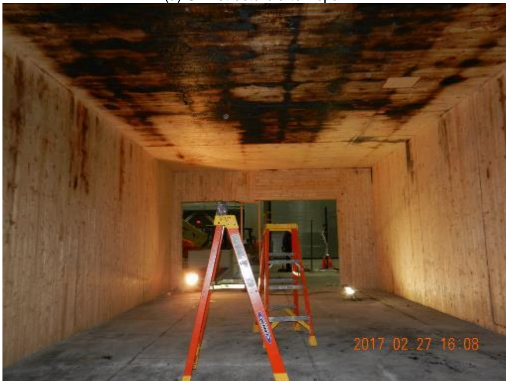
(b) CLT structure after repair
