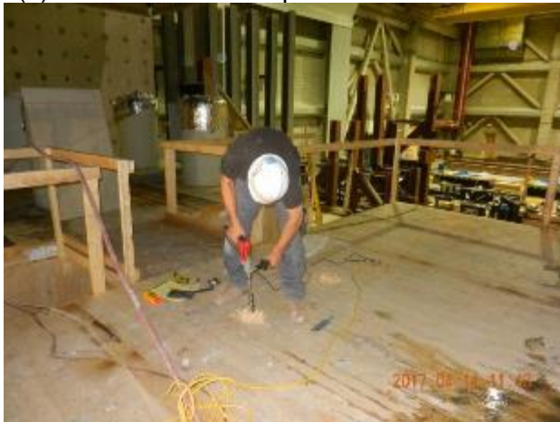
(c) drilling holes through ceiling panels
