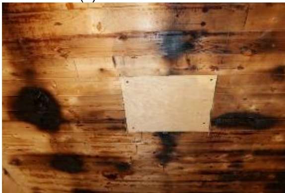
(c) plywood piece screwed in
